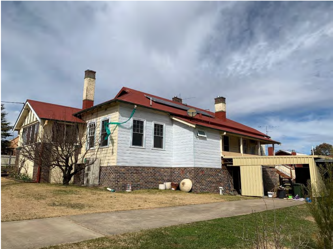
Image 5: North-west elevation viewed from King Street
