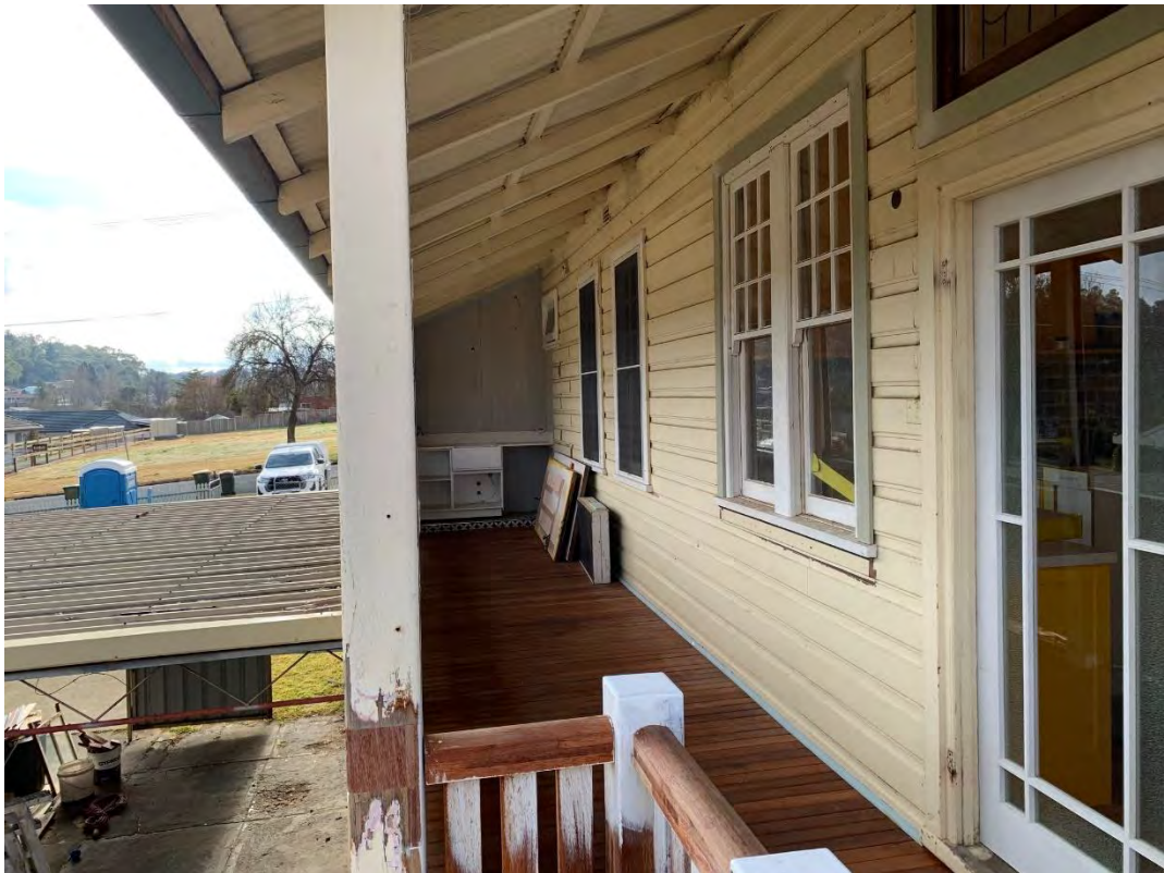
Image 10: Existing window and door openings to remain.
