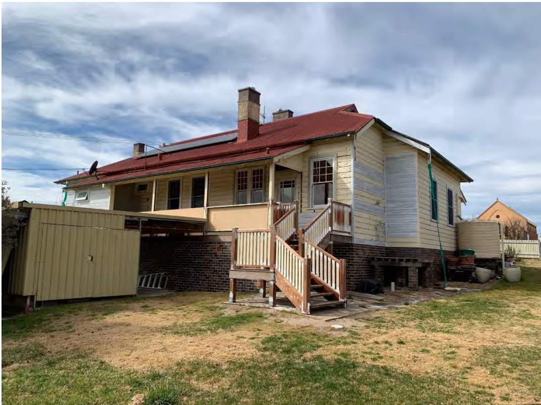
Image 6: North-west elevation viewed from property boundary adjoining 15 Bridge Street
