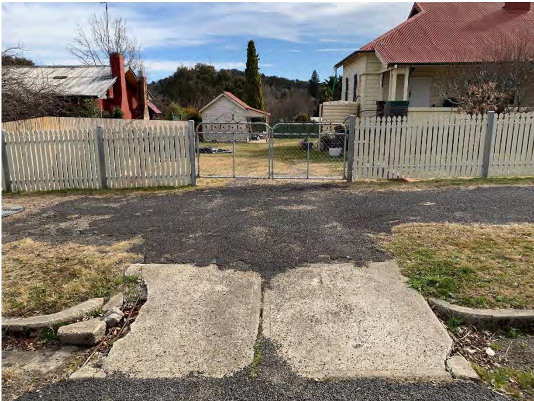
Image 8: Bridge Street vehicle entry. Entry gates and fence of metal posts and rails and timber pickets.
