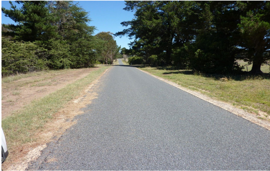
Figure 1.1: Condition Level 1 sealed road - Eastern Avenue, after rehabilitation
