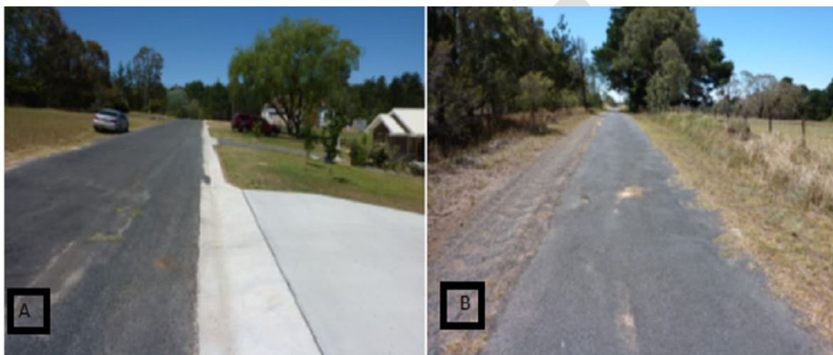
Figure 1.2: Photographs of (A) sealed road – condition 3 and (B) sealed road – condition 4.
