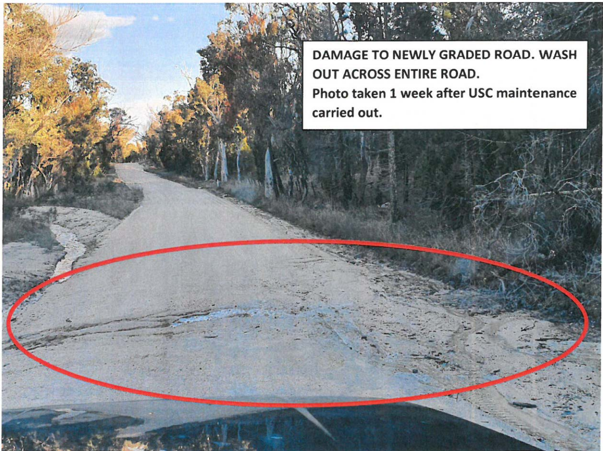
ROAD WASHING OUT AGAIN – SAME AREA AS PREVIOUS PHOTO Photo taken 1 day after reworks carried out (1 week after original maintenance.)
