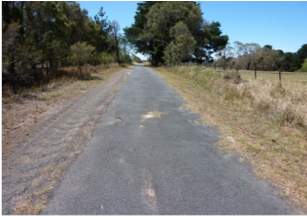
(e) Sealed Road – Condition 4 (Burtons Lane)
