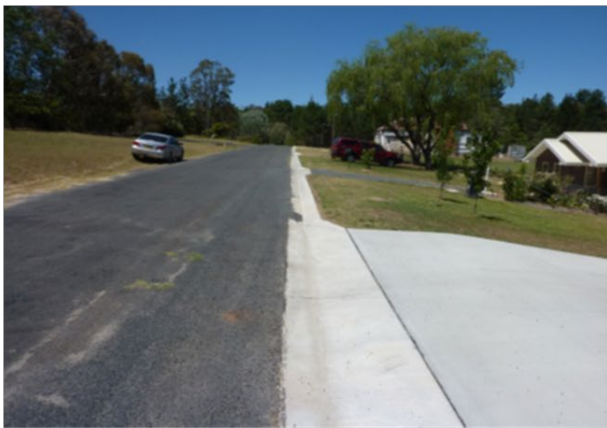
(g) Kerb and Guttering – condition 1 (Fitzroy Street)
