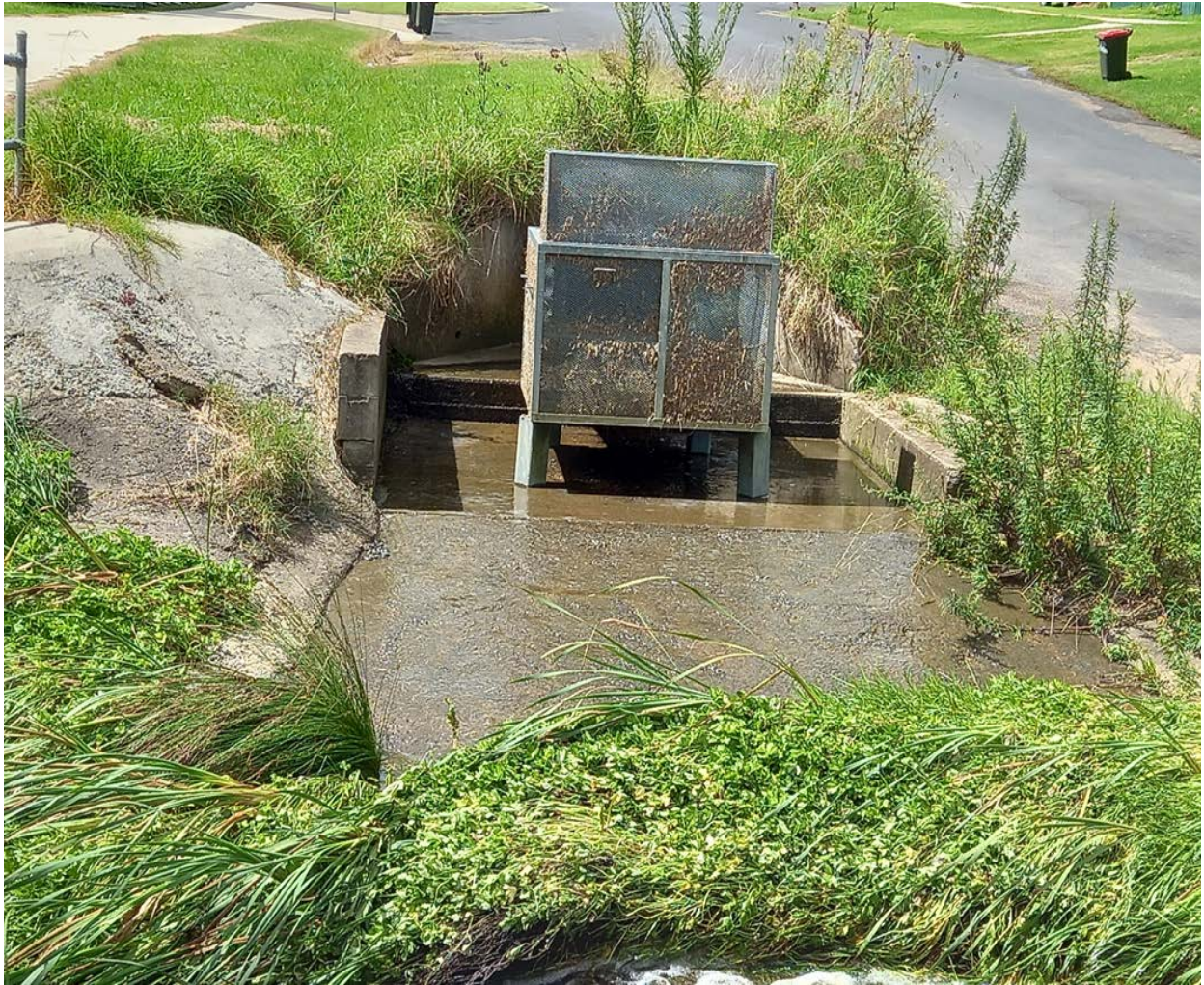
Figure 3.1: Gross Pollutant trap in condition 1
