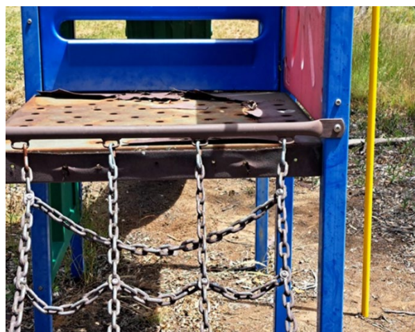
Obsolete playing equipment and worn-out protective coating of metallic stand behind Grace Munro Aged Care Centre in Bundarra
