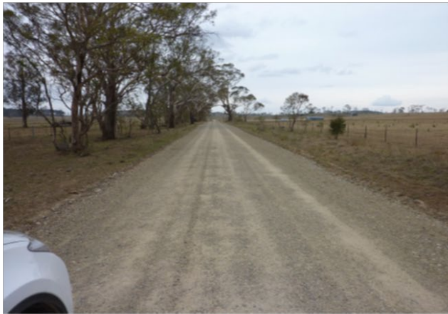
(c) Unsealed Road – service level (Big Ridge Road)
