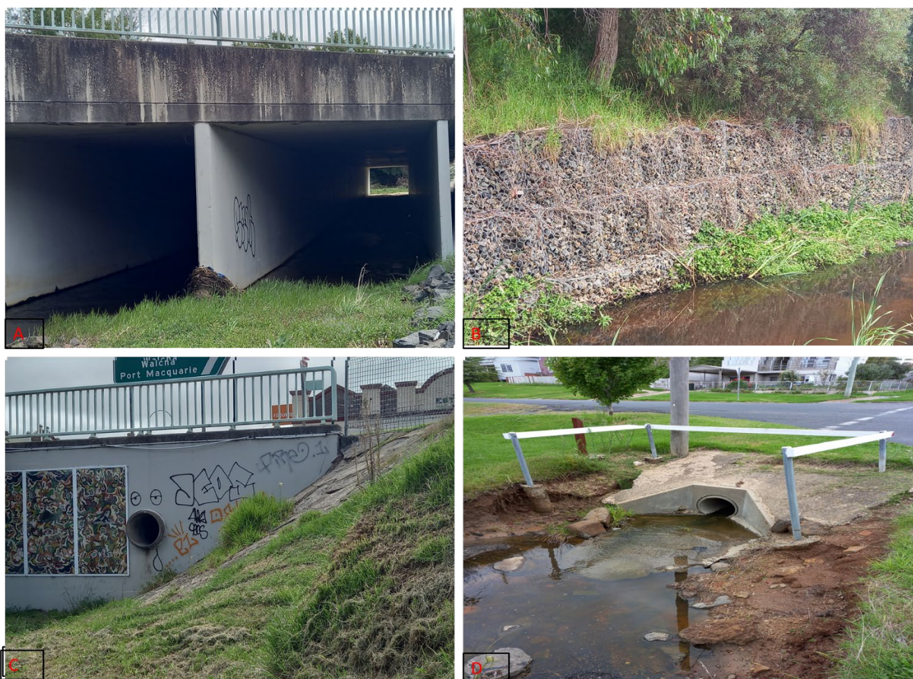
Figure 5.1 Examples of stormwater assets (A) Box culvert, (B) Waterway gabion protection (C) and (D) Pipes.
