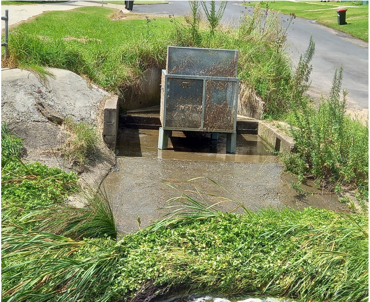
Figure 3.1: Gross Pollutant trap in condition 1
