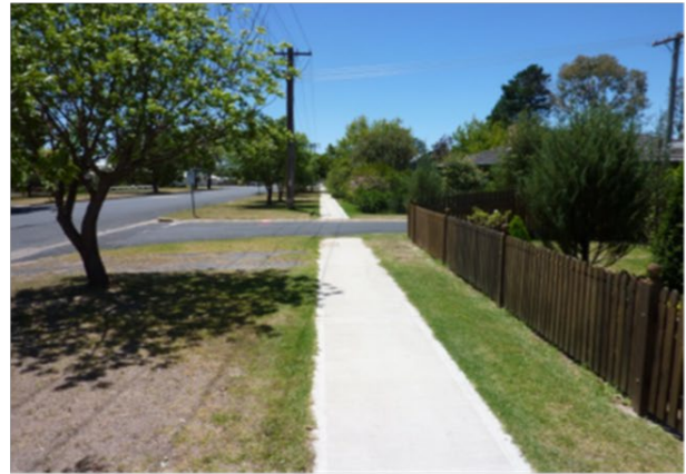
(h) Footpath – Condition 1 (John street)
