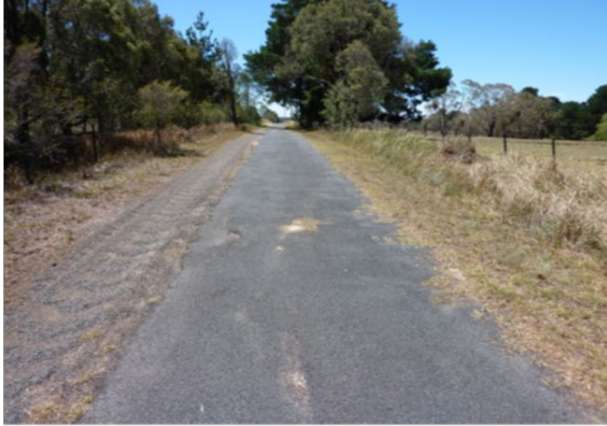
(e) Sealed Road – Condition 4 (Burtons Lane)
