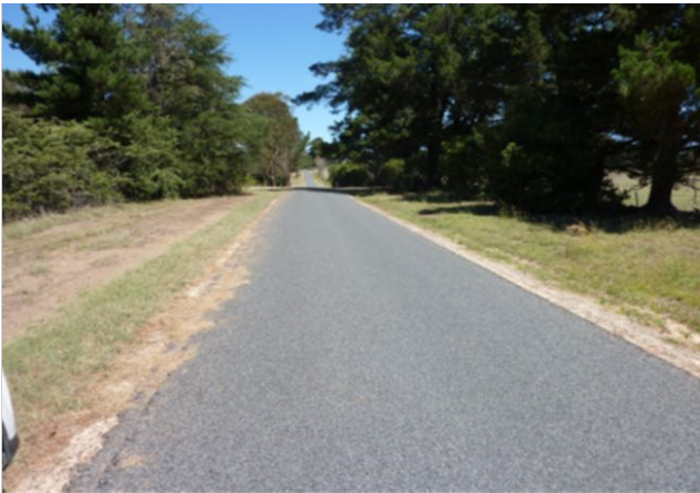
(a) Sealed Road – Condition 1 (Eastern Avenue)
