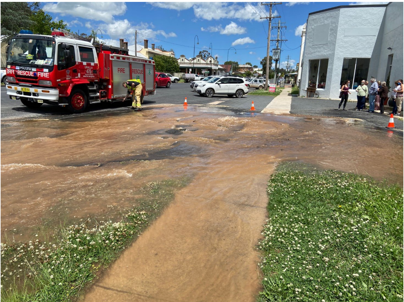
Figure 5-2 - Burst trunk main in Hill Street, Uralla (2021)
