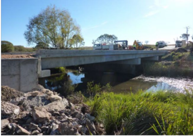
(i) Concrete Bridge replacing a timber bridge – Enmore Road,
