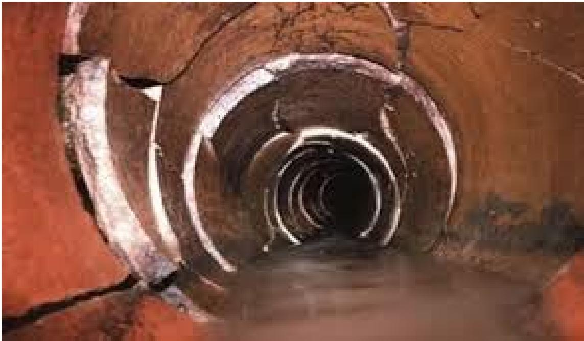
Figure 5.1.2. Example image of a badly broken sewer pipe inspected with CCTV
