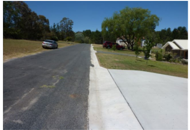
(b) Sealed Road – Condition 3 (Fitzroy Street)
