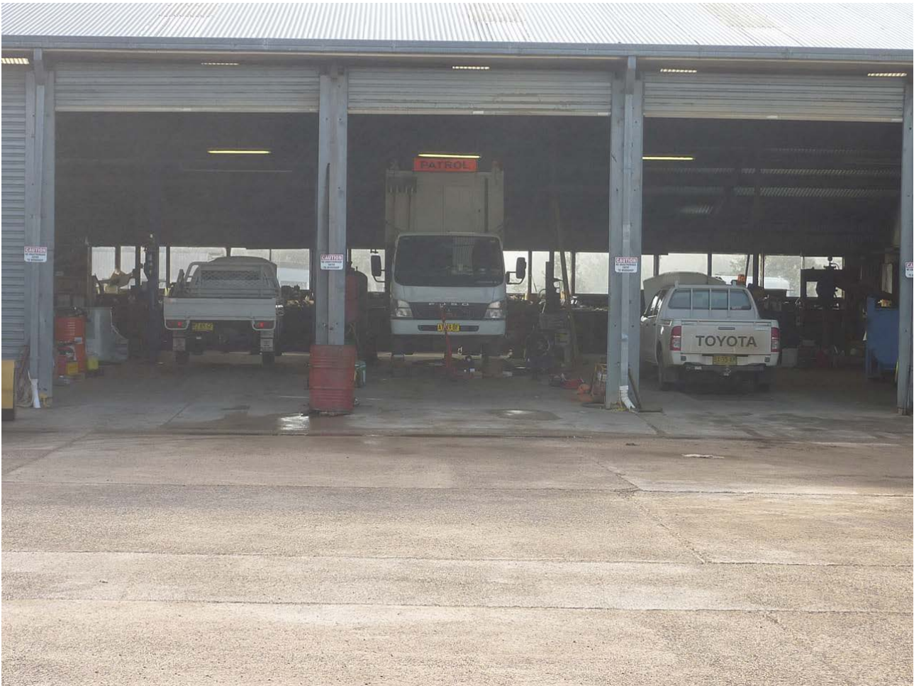
Figure 4–Uralla Shire Council Workshop – Uralla Depot
