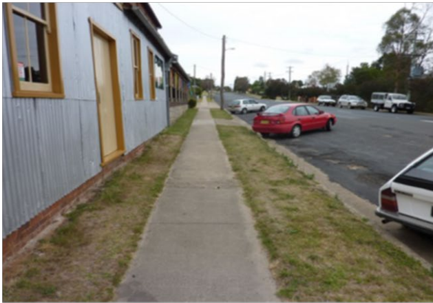
(k) Footpath – Condition 3 (Salisbury Street)
