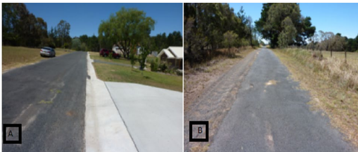
Figure 1.3: Photographs of (A) sealed road – condition 3 and (B) sealed road – condition 4.
