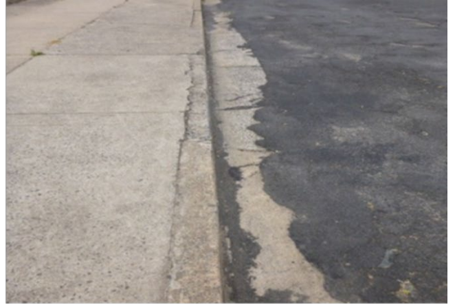
(j) Kerb and Guttering – Condition 3 (Salisbury Street)
