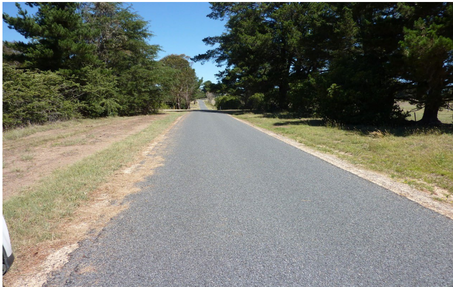
Figure 1.2: Condition Level 1 sealed road - Eastern Avenue, after rehabilitation
