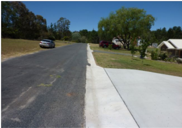
(g) Kerb and Guttering – condition 1 (Fitzroy Street)
