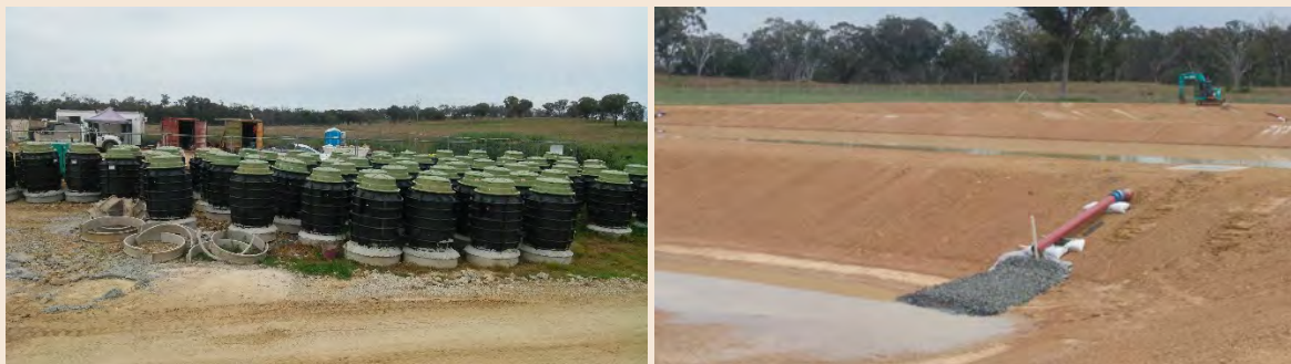
Figure 3: Ongoing construction works and equipment at the Bundarra Sewage Treatment Plant
