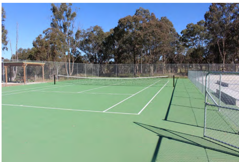
1 Bundarra Multi-Purpose Courts
