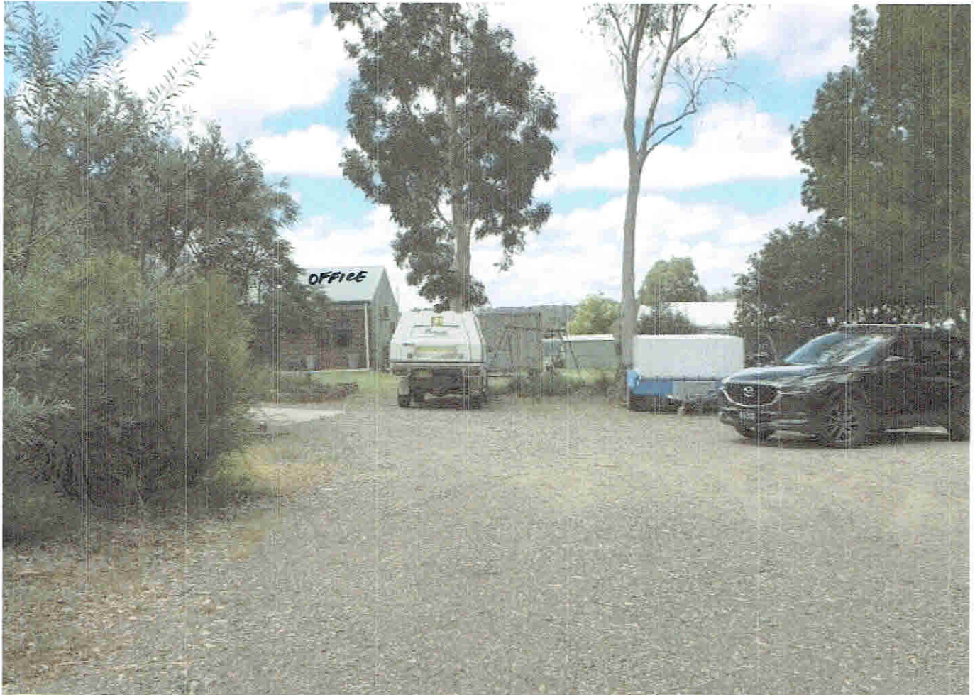
VIEW OF EXISTING OFFICE FROM ENTRANCE DRIVEWAY.
