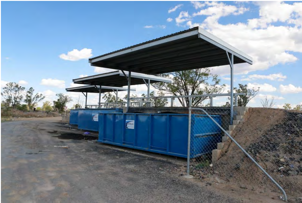
Figure 3-1 RORO Bin Transfer Station in Saw-Tooth Configuration
