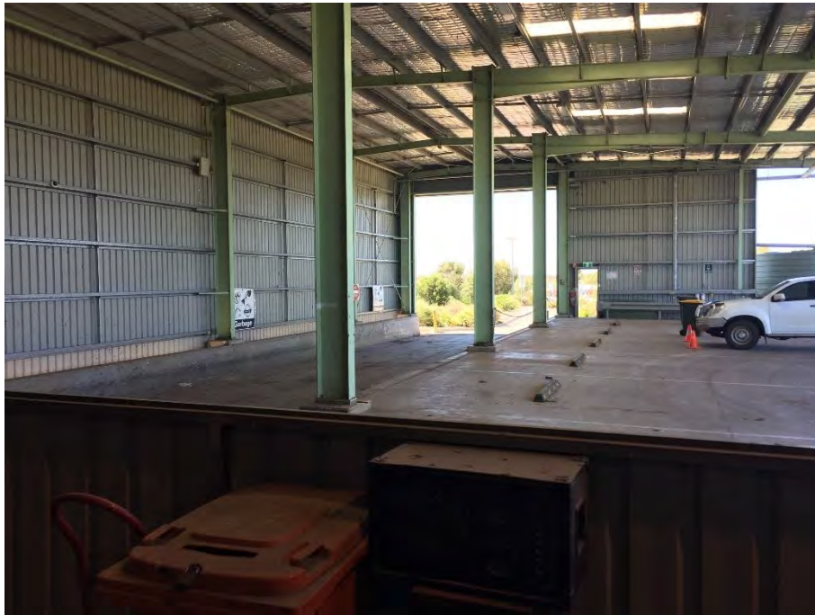
Figure 3-2 Example of Flat Floor Transfer Station
