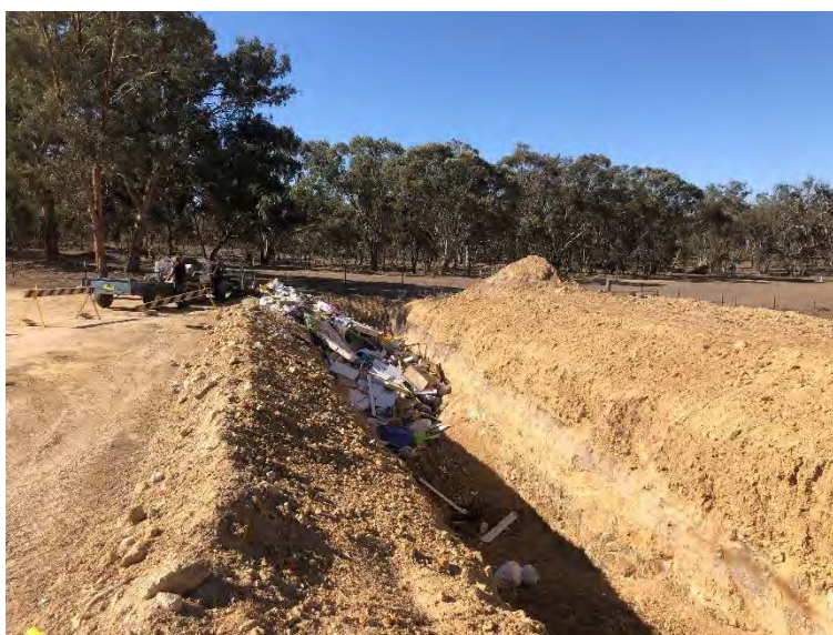
Figure 2-6 Current Landfill Cell – Bundarra Waste Facility
