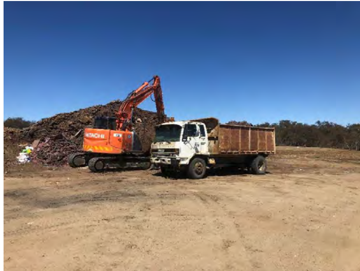
Figure 2-7 USC 12T Excavator and 8T Truck
