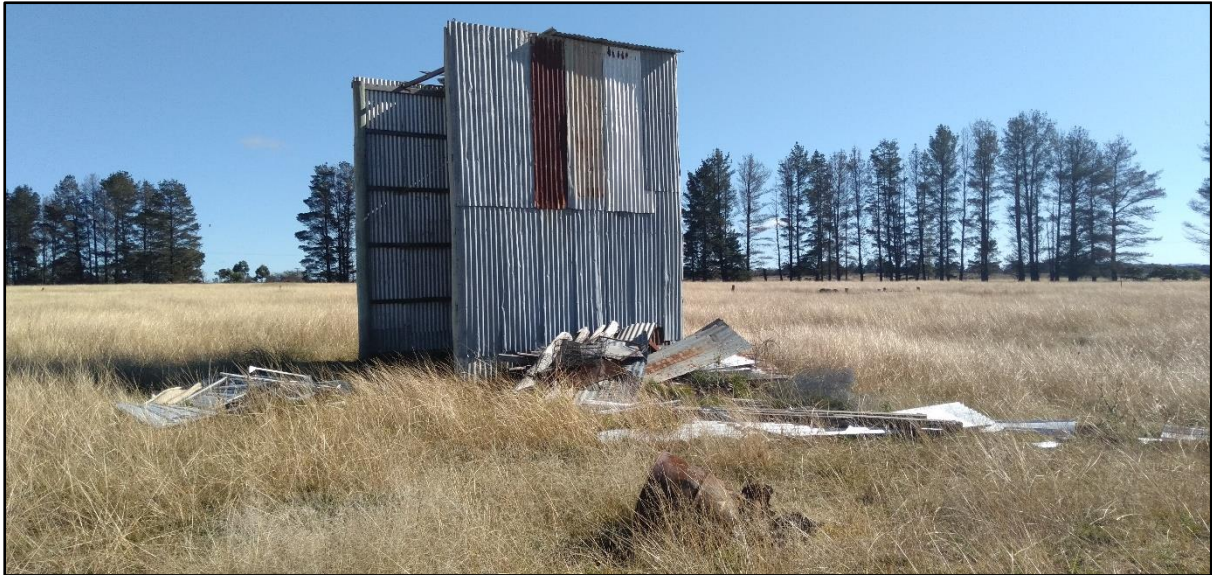
Figure 16: Existing dilapidated building on property (to be removed), view facing north.
