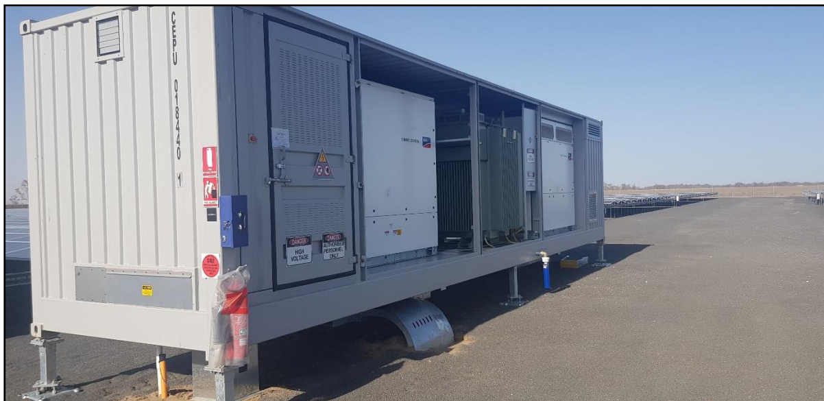
Figure 6: MVPS Skid and Inverter
