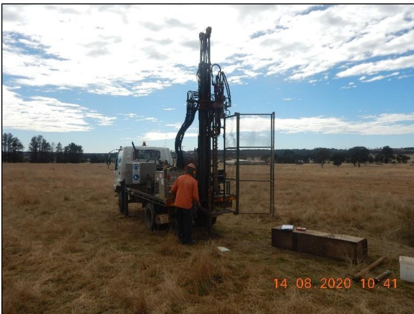
Figure 2: Drilling rig on Bore 2 location
