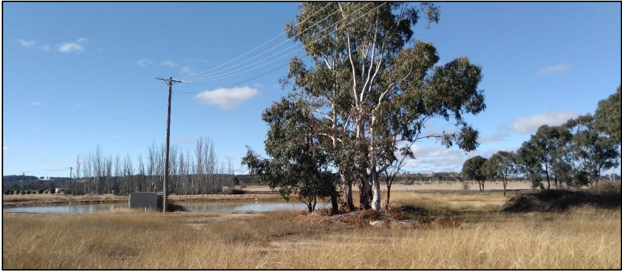
Figure 19: Existing storage, powerlines and structures on the property, view facing north-east.
