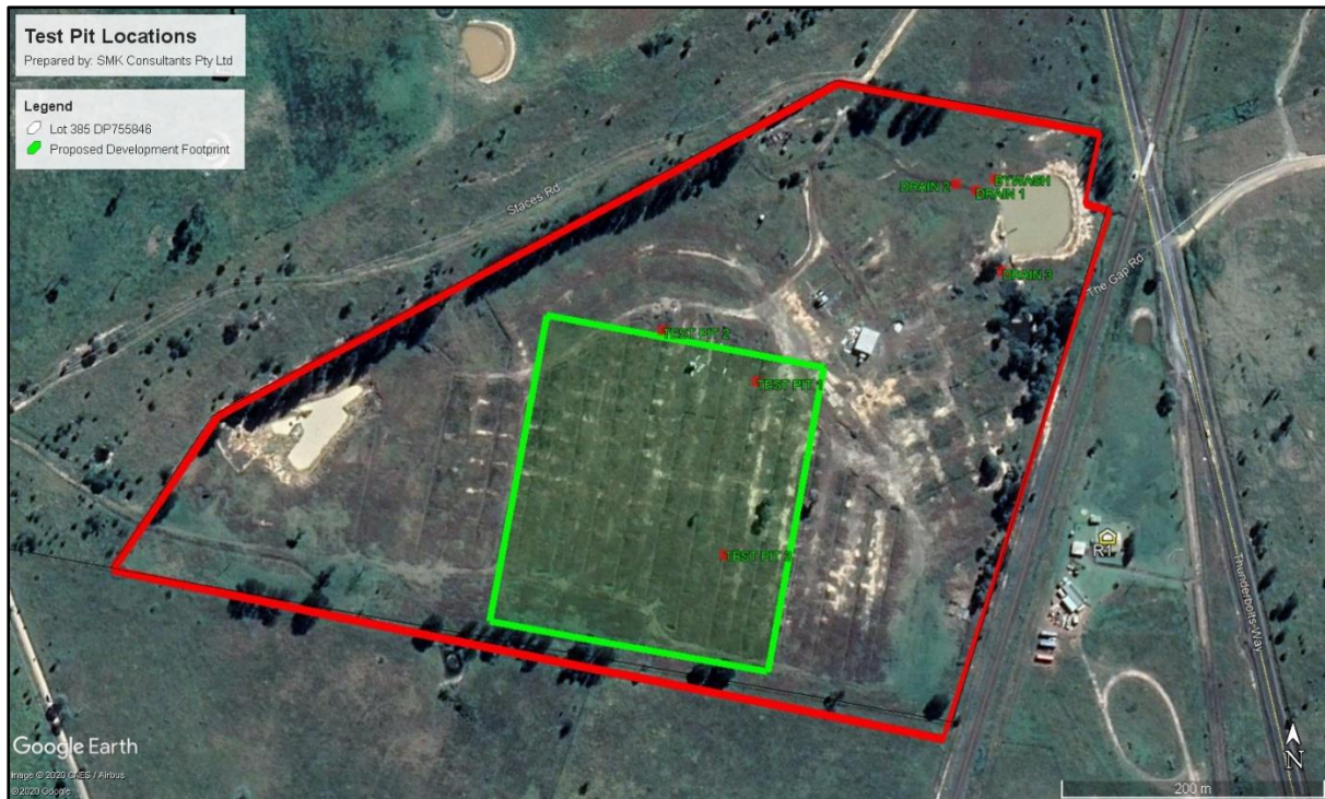
Figure 1: Test Pit Locations
