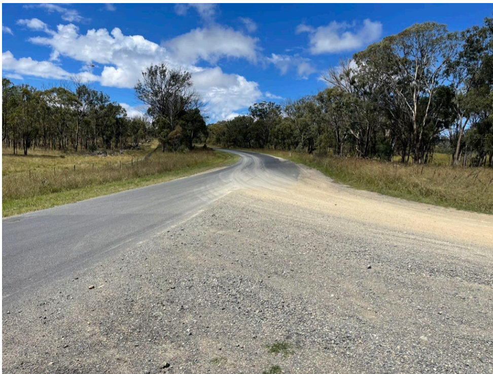
Figure 6-13: Carlon's Quarry access road intersection looking east
