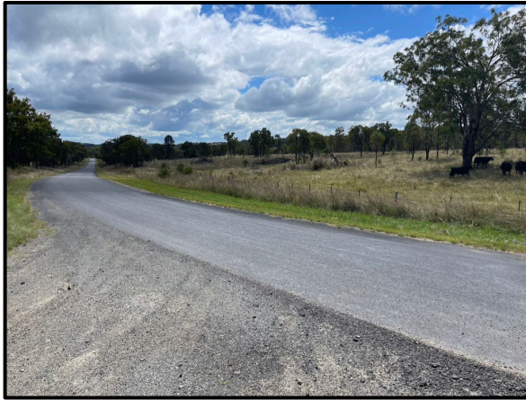
Plate 7 - Carlton's Quarry Access Road looking west
