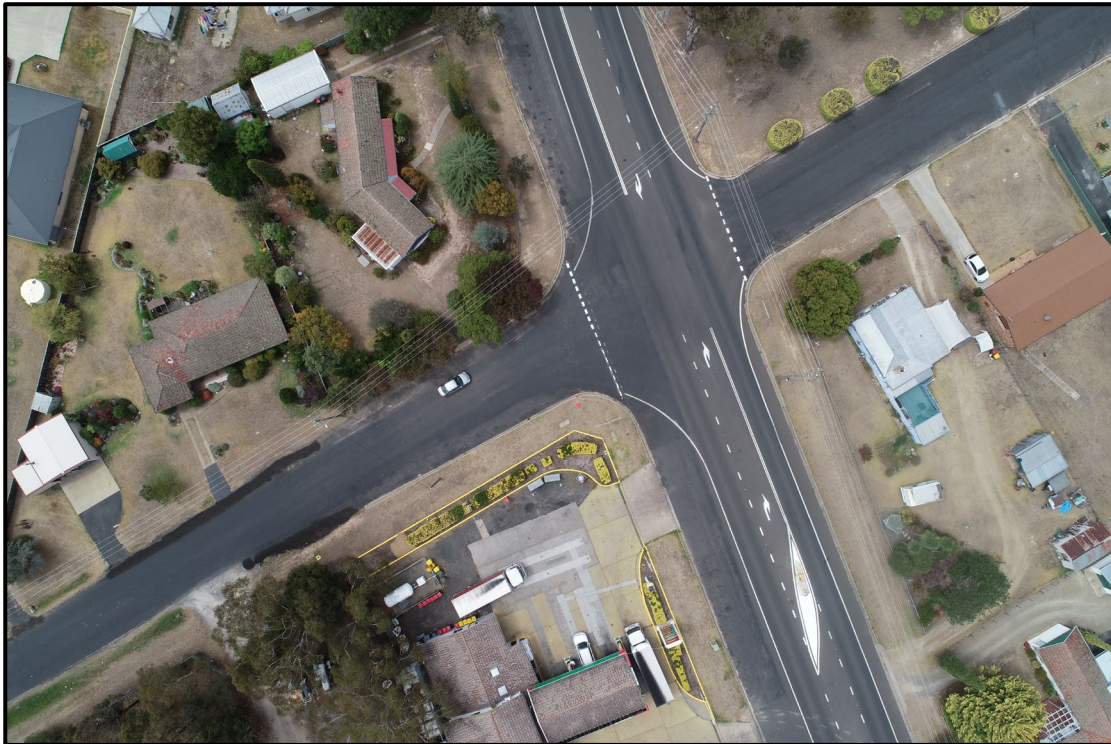
Plate 9 – Kingstown Road (East Street) Intersection with the New England Highway
