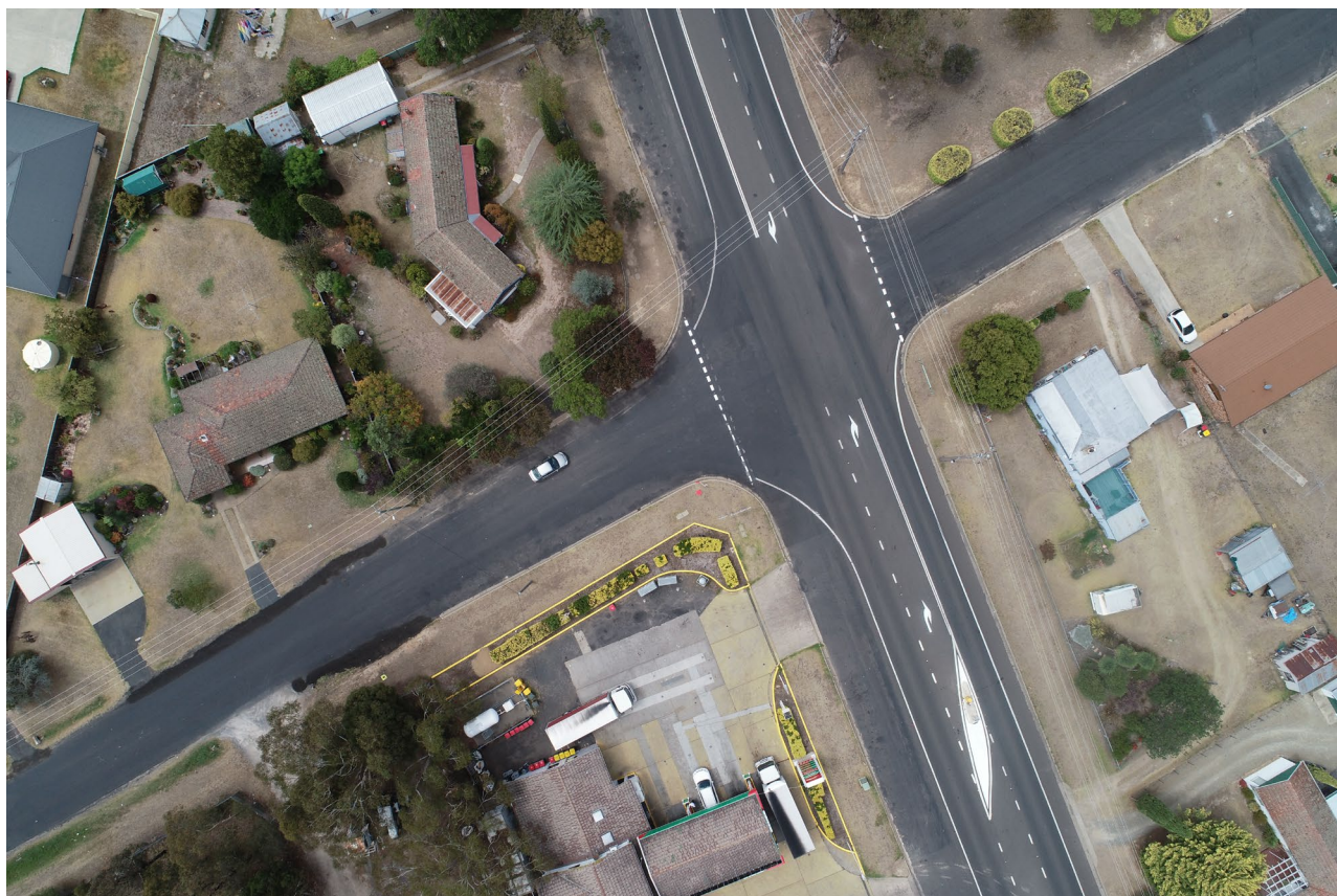
Figure 6-14: Kingstown Road (East Street) intersection with the New England Highway
