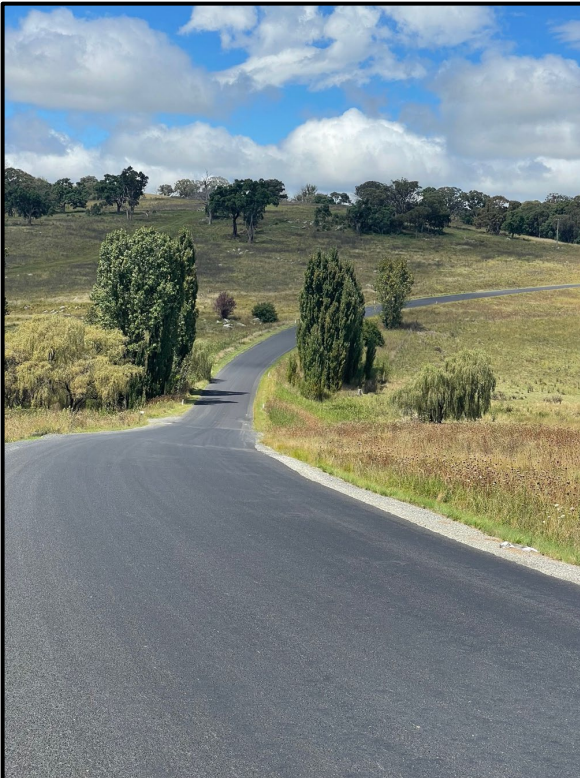
Plate 3 – Kingstown Road 7.5km from the Highway looking east
