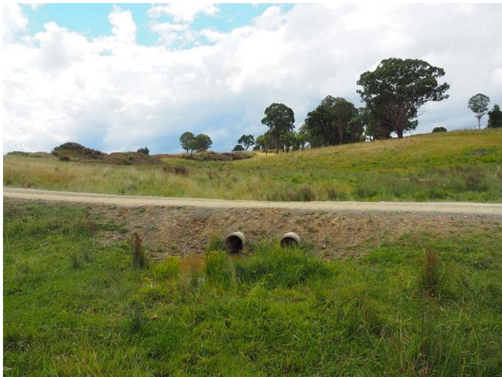
Figure 3.9 - Existing culvert crossing at the access road to the quarry
