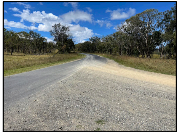
Plate 8 - Carlton's Quarry Access Road looking east
