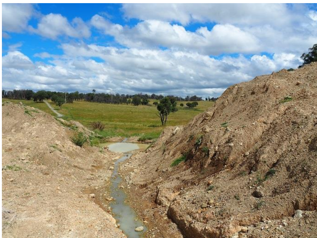
Figure 3.8 - Ground surface conditions at lower areas of the quarry near the sediment pond
