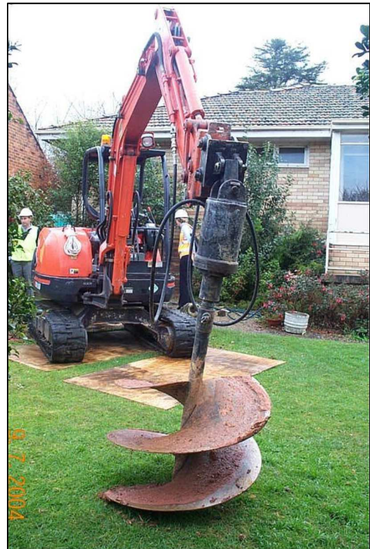
Typical Excavation for Low Pressure Pump Unit
