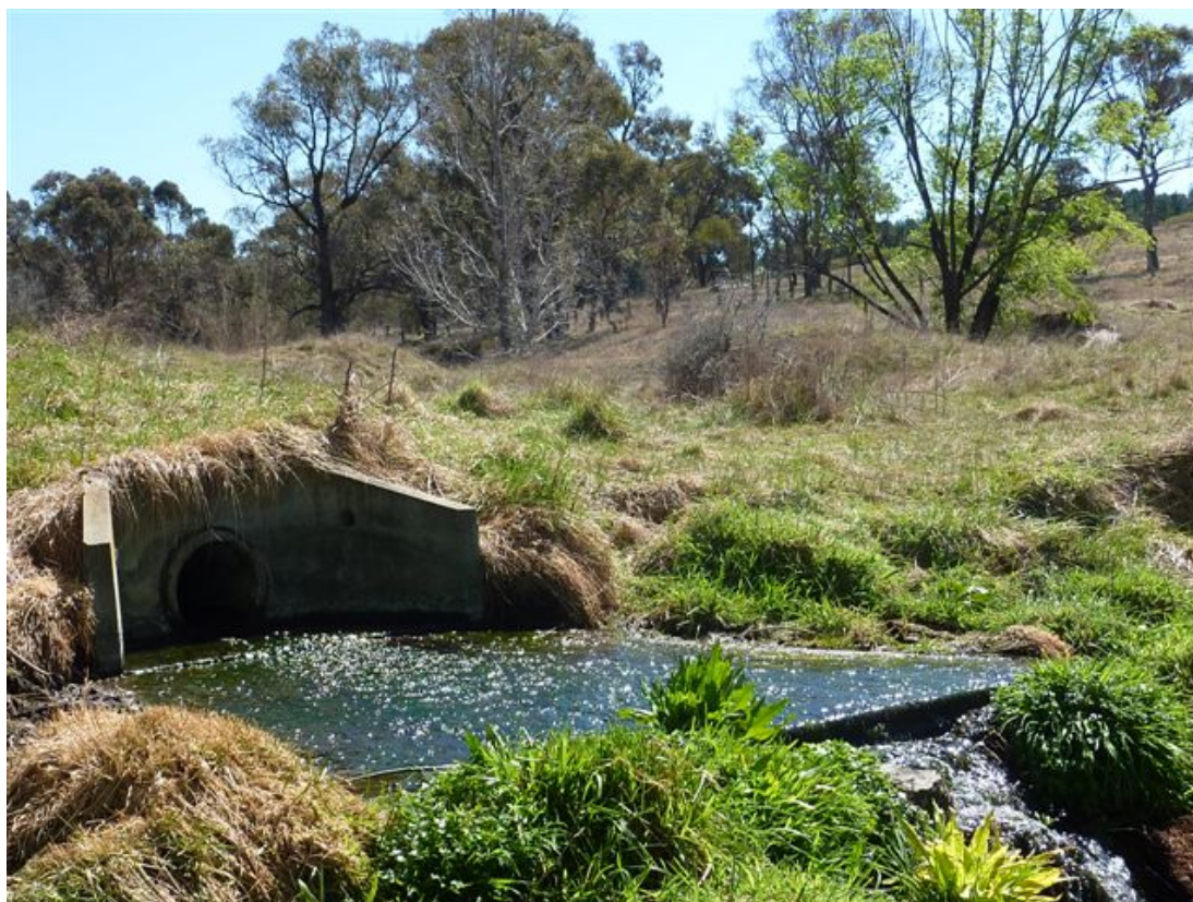
Figure 3.3 Outflow from plant into Chinamans Gully.
