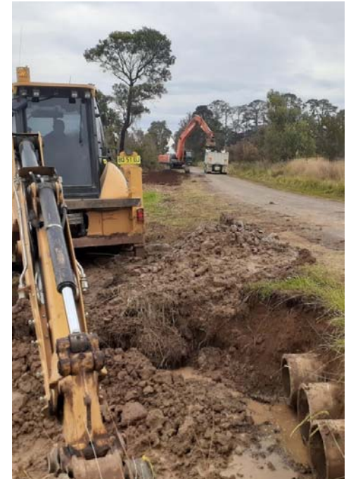
Drainage works Hawthorne Drive Arding
