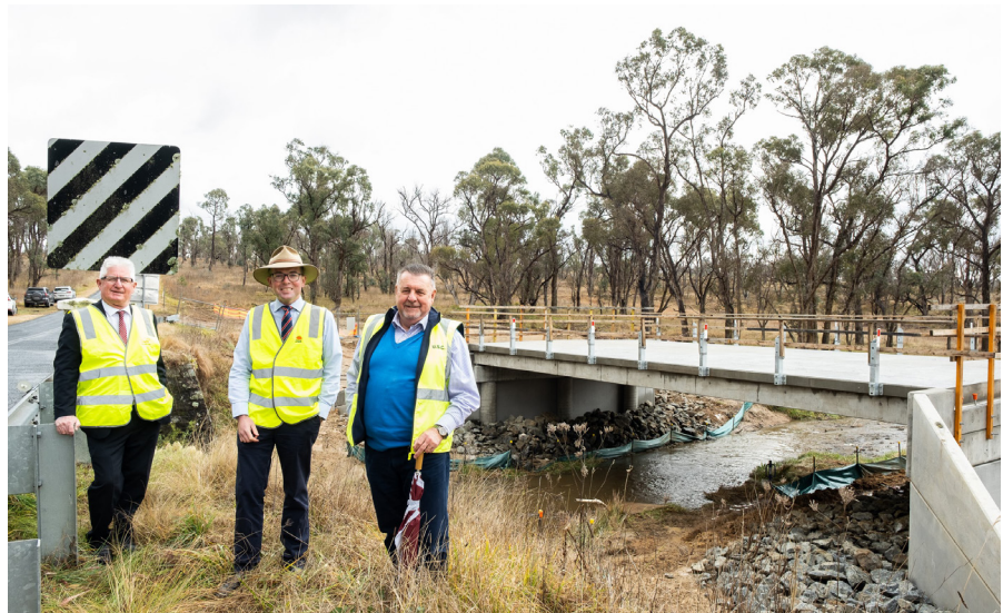
Inspecting construction of the new Tolleys Gully Bridge: L-R Terry Seymour (USC Director Infrastructure & Development), Adam Marshall MP and Mayor Michael Pearce
