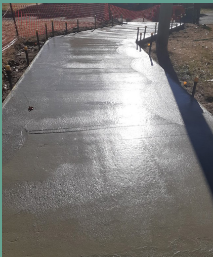
Plane Ave shared path construction
