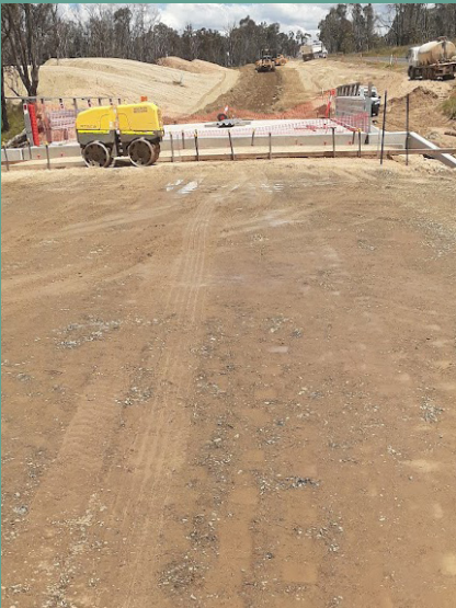
Constructing approaches to Tolleys Gully Bridge
