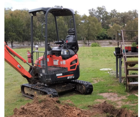
Pictured: Work continues on connecting a house in Bowline Street, Bundarra despite the Gwydir River running to the top of the bank.
