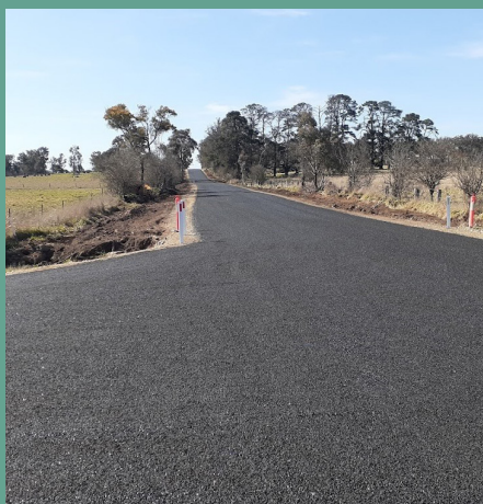
Stage 1 of Hawthorne Drive has been completed
