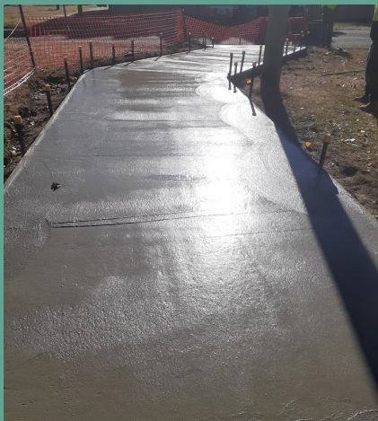
Plane Ave shared path construction
