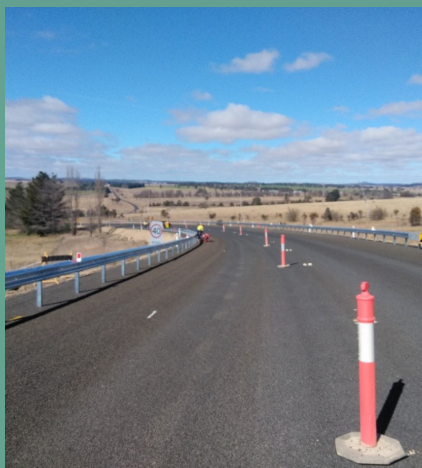
Installing safety rail on the Tarana Curve
