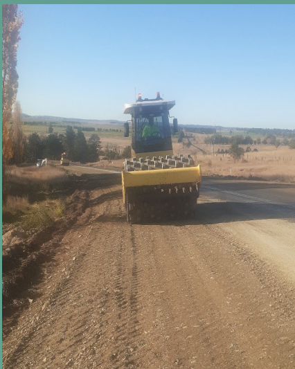
Thunderbolts Way (MR73) Tarana curve construction
