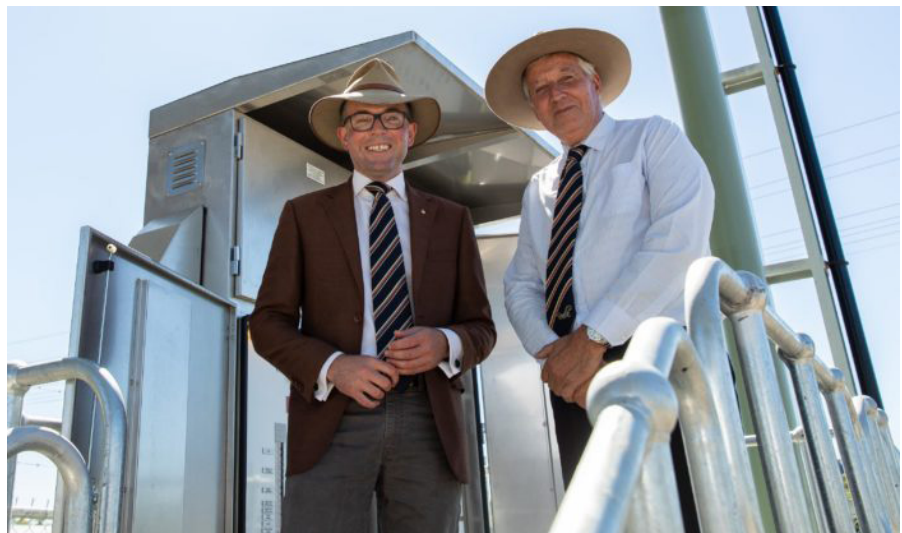
Adam Marshall MP and Mayor Robert Bell 'flick the switch' on the new $8.8 million Bundarra Sewerage Scheme Project (photo c/ Adam Marshall's office)
