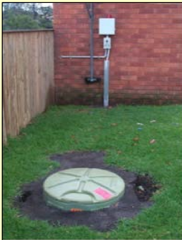
Pod and switchboard arrangement
