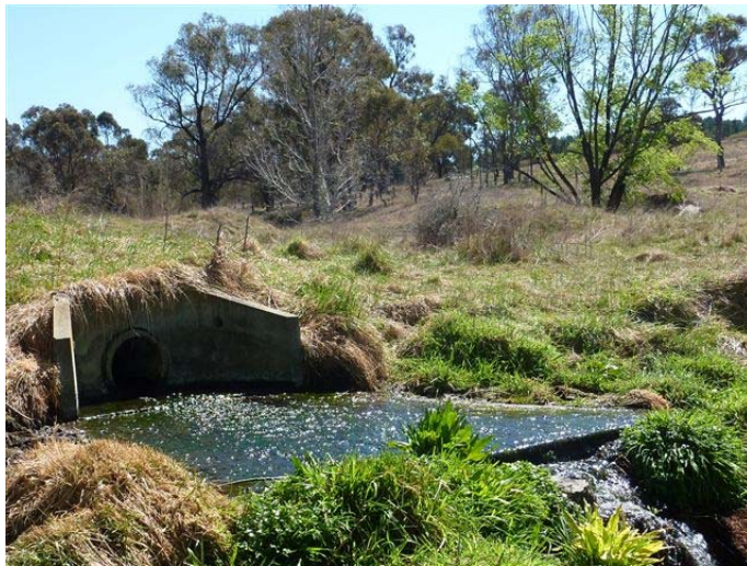
Figure 3-3 Outflow from plant into Chinamans Gully
