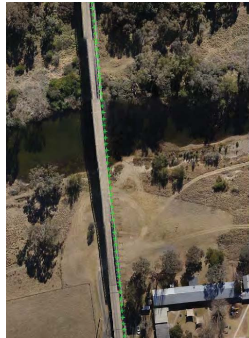
Pipeline Bridge Crossing Alignment
