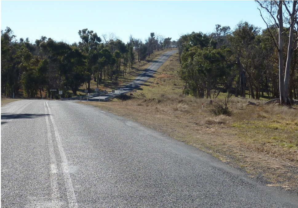
Photo 3. Approaches to Bridge looking west towards Bundarra. It is proposed that the new bridge will be located on a straighter alignment to the right (downstream) of the existing bridge. Full design plans for the approaches have been prepared.
