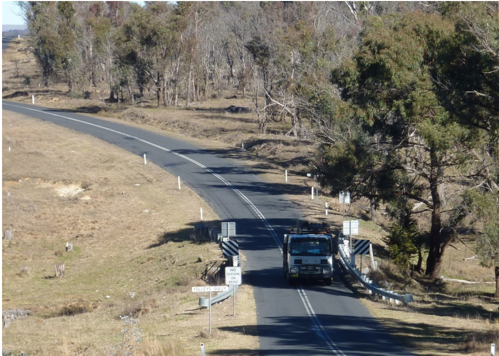
Photo 1. Looking east towards Uralla. Note the narrow bridge width which B-double trucks will need to negotiate when the route is opened to HML vehicles.
