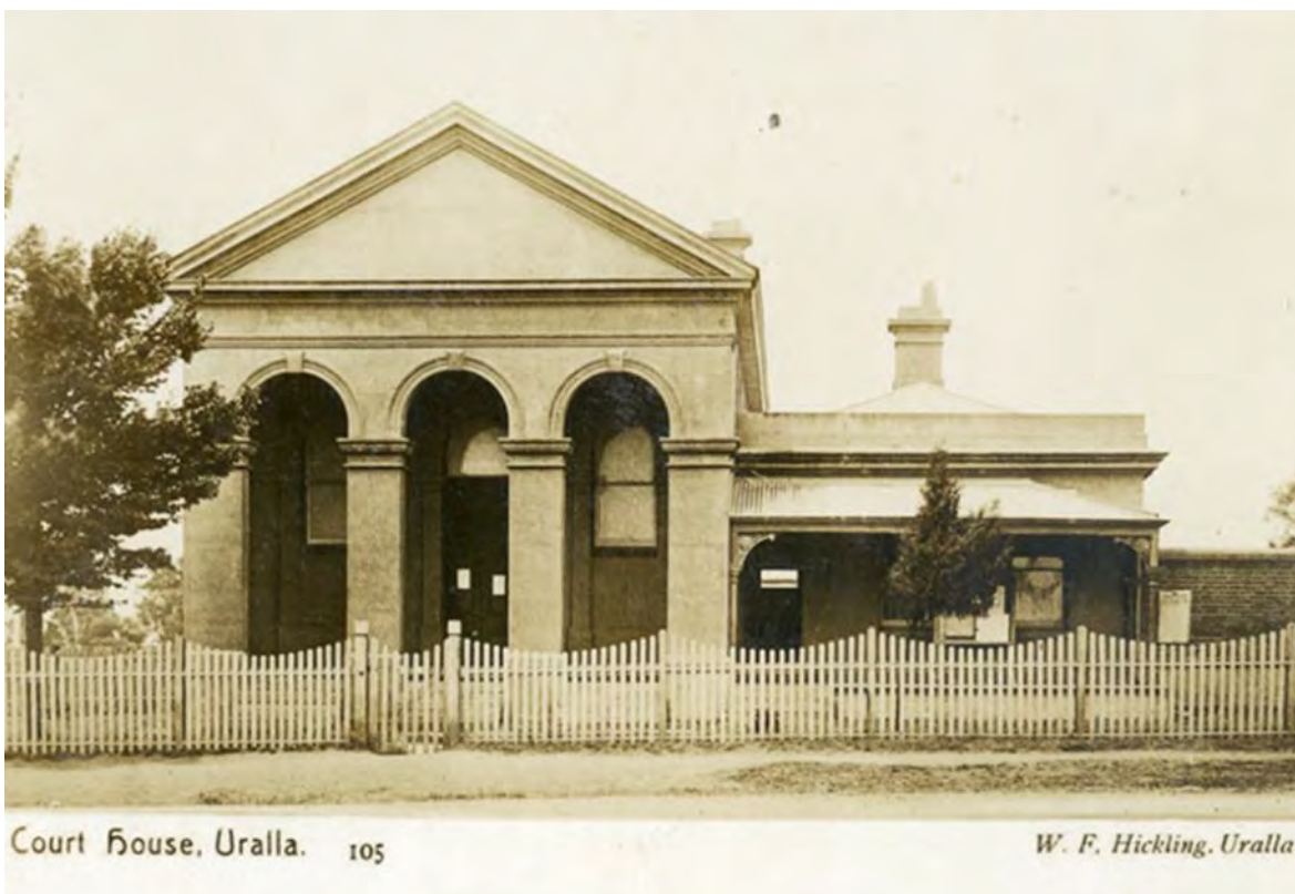
Undated image of former Court House (Hill St)
