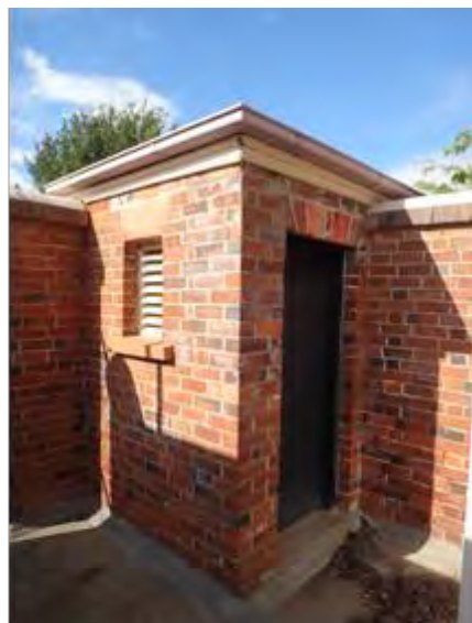
Typical external toilet
