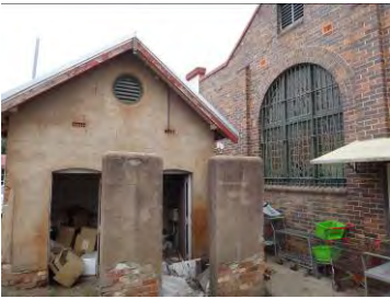
partially detached toilet block
