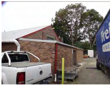
attached skillion storage area
