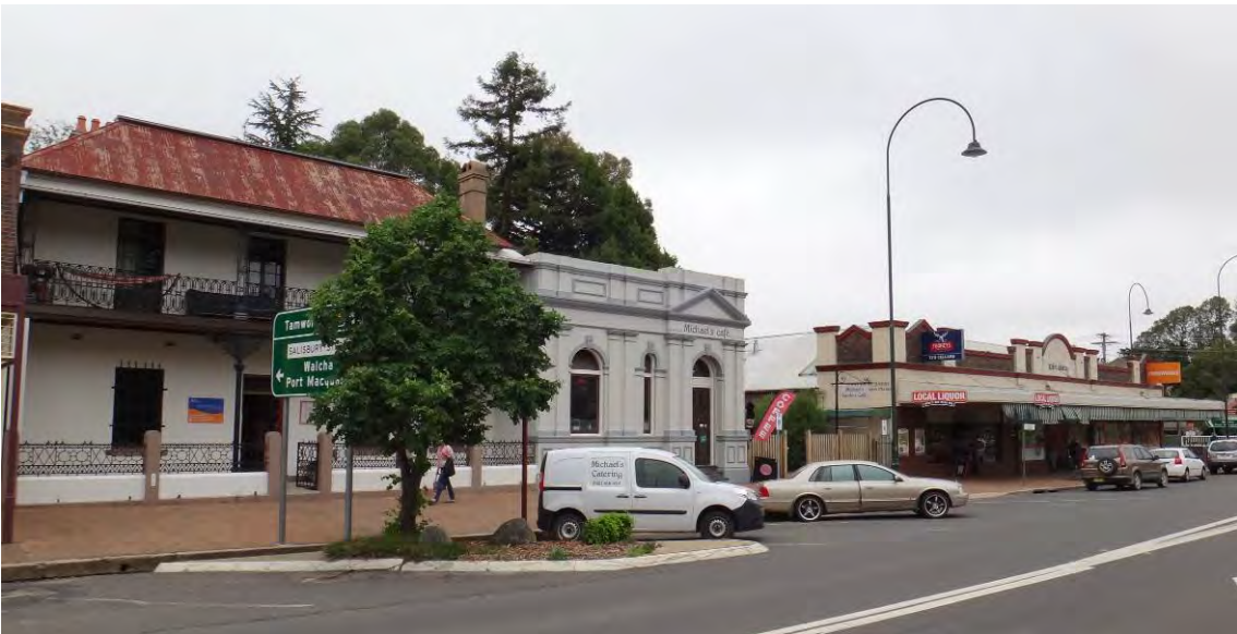
Image: View looking south along Bridge Street from former Bank of NSW which adjoins Foodworks The existing building is on a corner location and prominent within the Uralla streetscape with an interesting parapet and roof form and lead lighting over several windows.
