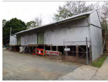
metal clad shed
