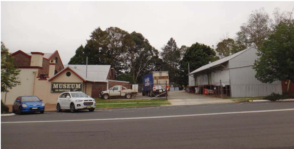
Images: Salisbury Street frontage showing three buildings proposed to be demolished.
