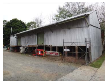
metal clad shed
