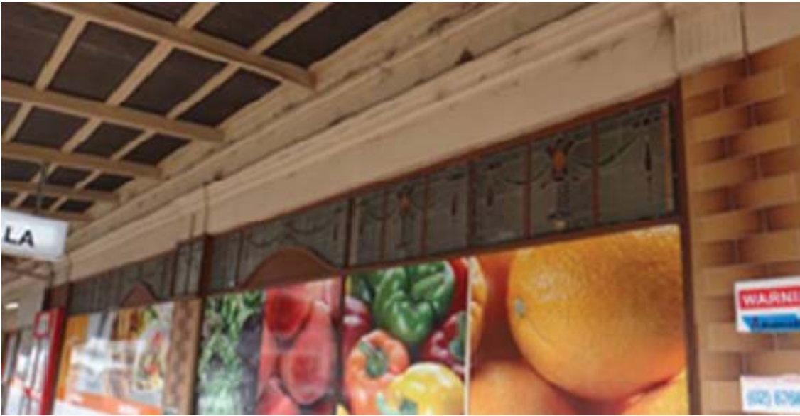
Image: Lead light over windows Bridge Street frontage.
