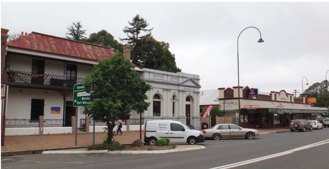
Image: View looking south along Bridge Street from former Bank of NSW which adjoins Foodworks The existing building is on a corner location and prominent within the Uralla streetscape with an interesting parapet and roof form and lead lighting over several windows.
