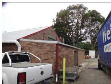
attached skillion storage area
