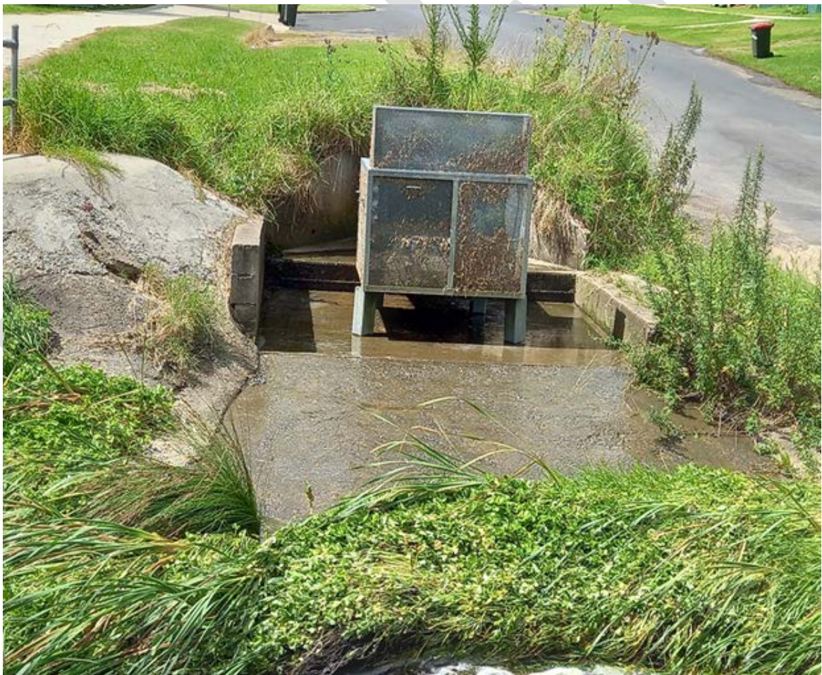
Figure 3.12.2: Gross Pollutant trap in “Excellent” condition
