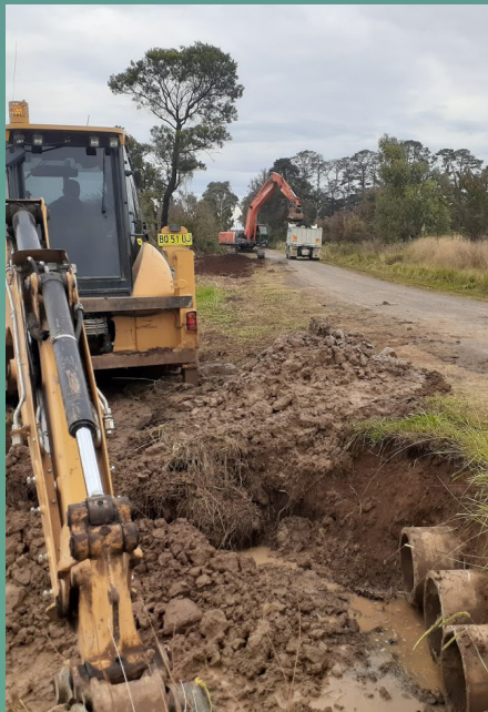
Drainage works completed on Hawthorne Drive, Arding.
