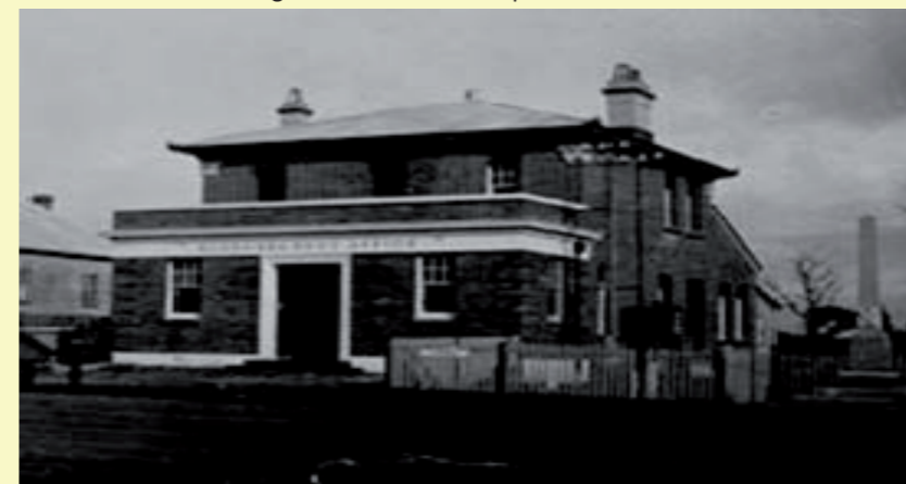
PHOTO BELOW: Showing the 1930's Brick Parapet structure
