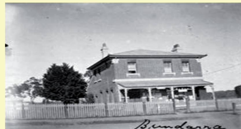
PHOTO ABOVE: Pre 1930's with open verandah
