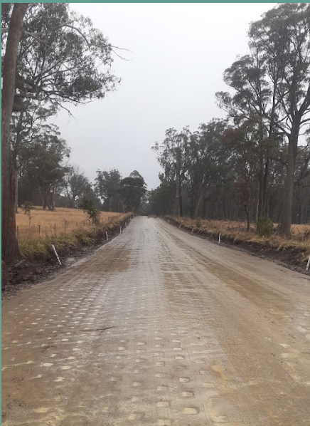
Hawthorne Drive Stage 2 Construction
