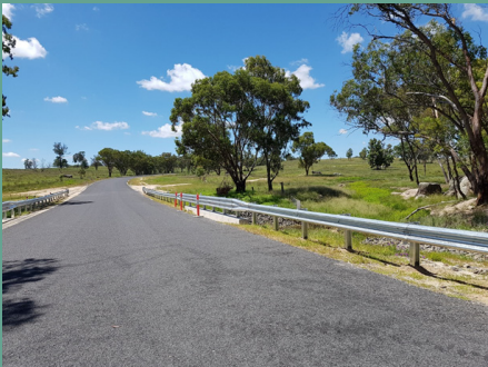
Completed guard rail installation on Myall Swamp Bridge - Bingara Road Construction
