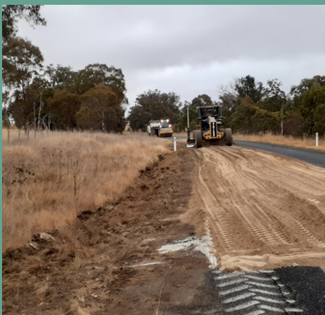
Heavy Patching on Kingstown Road
