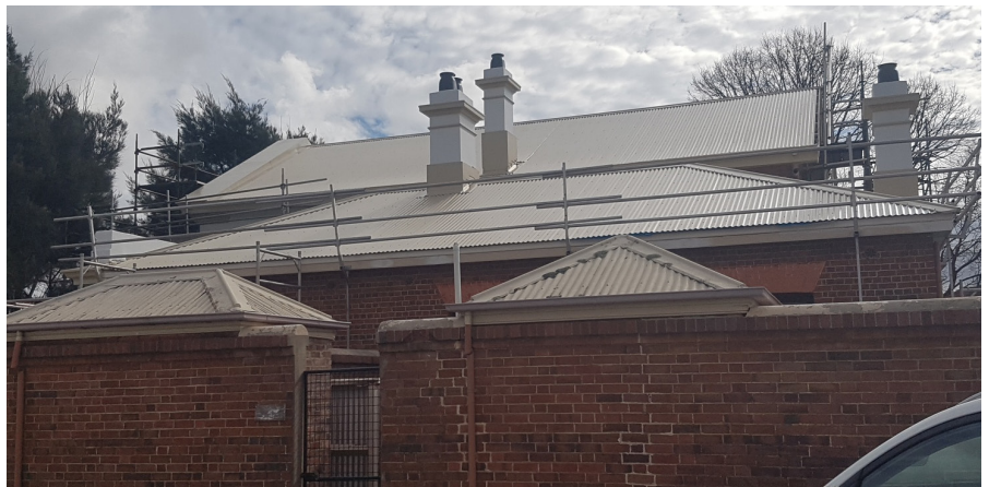
New roofing on the Uralla Court House has been completed. One of Council's projects in the adopted Delivery Program 2022-2026 is to develop the Old Court House as a community entertainment venue.
