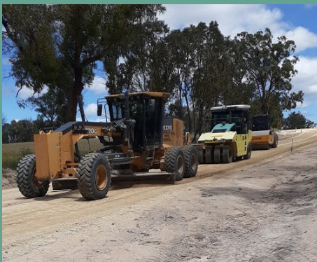
Retreat Road upgrade.
