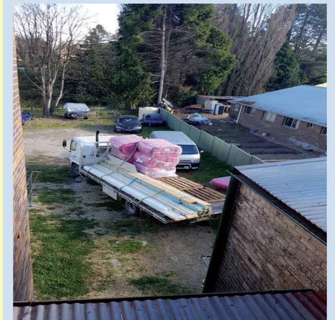
Photo: Delivery of the insulation.
