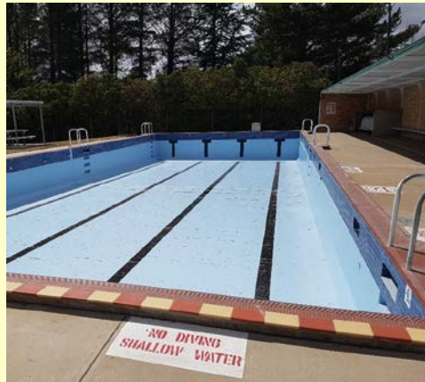
Resurfacing of the pool completed during the month of September 2019.
