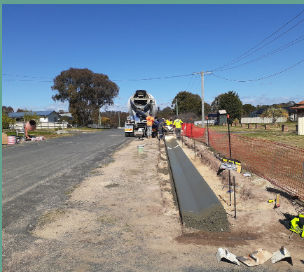
Kerb and gutter works underway at Roman Street, Uralla
