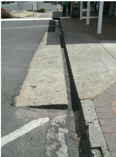
Fig 18 & 19. Gaps or channel left in driveways, while achieve vehicle crossing: They restrict flows and provide a risk to pedestrians. In detail design, consider using a porous 10mm aggregate no-fines concrete driveway ramps. – While not highly durable it can be easily repaired, unlike concrete.
