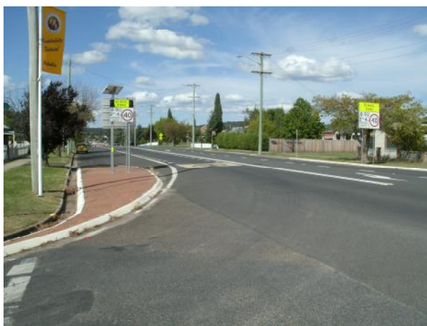
Fig 8. (duplicate of Fig 7) shows Closed in intersection, with no double kerb and landscaping. This visually encloses the intersection slowing traffic.
