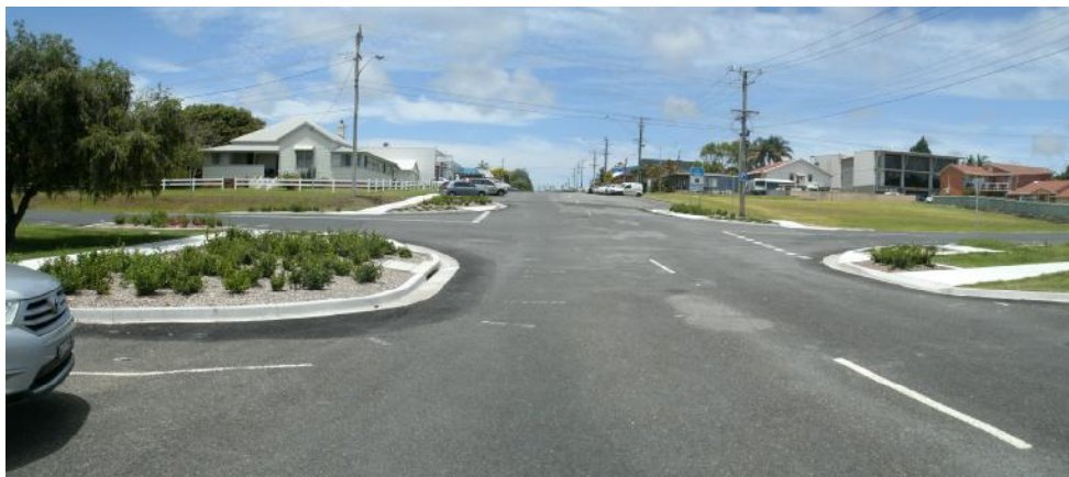
Fig 8. (duplicate of Fig 7) shows Closed in intersection, with no double kerb and landscaping. This visually encloses the intersection slowing traffic.
