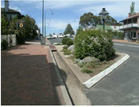
Fig 12. One of the larger planting islands where the driveway is seldom used, with no trees to act as laterals and rocks and tall shrub planting restricting sight-lines. Additionally, the island is bordered by excessive paving, which restricts water and air supply to root systems.
