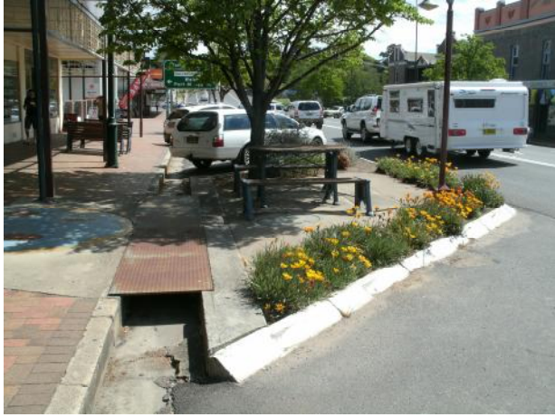
Fig 16 & 17. Street Tree Planting islands encroached by paving and typical existing double kerb drainage with metal plate cover appears like an after thought or solution that does not integrate with the streetscape.
