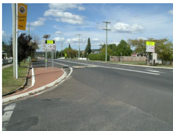
Fig 21 & 22. Street and traffic signage needing relocation towards the traffic lanes, with the Closed-in intersection kerb lines
