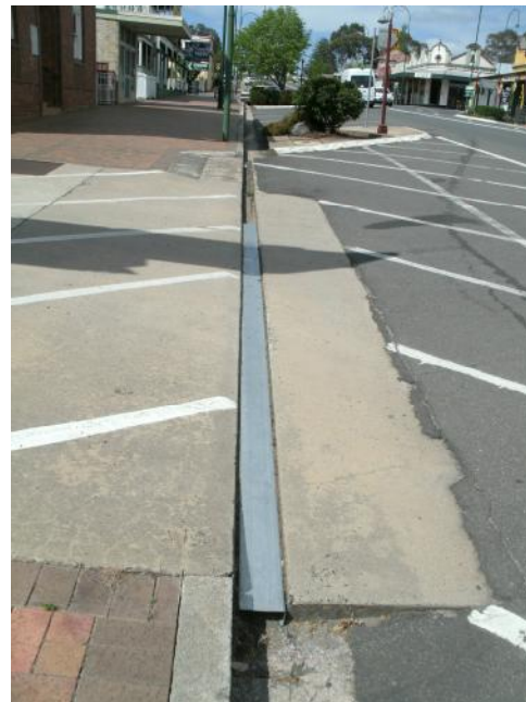
Fig 18 & 19. Gaps or channel left in driveways, while achieve vehicle crossing: They restrict flows and provide a risk to pedestrians. In detail design, consider using a porous 10mm aggregate no-fines concrete driveway ramps. – While not highly durable it can be easily repaired, unlike concrete.
