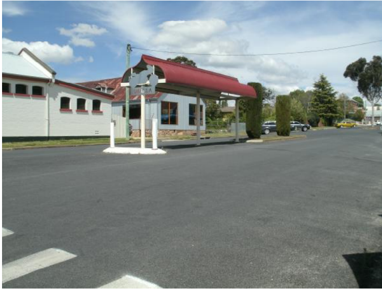
Fig 3. East Hill Street: Motorcycle parking and landscape median, lends itself to pedestrian refuge. - With or without a marked crossing.
