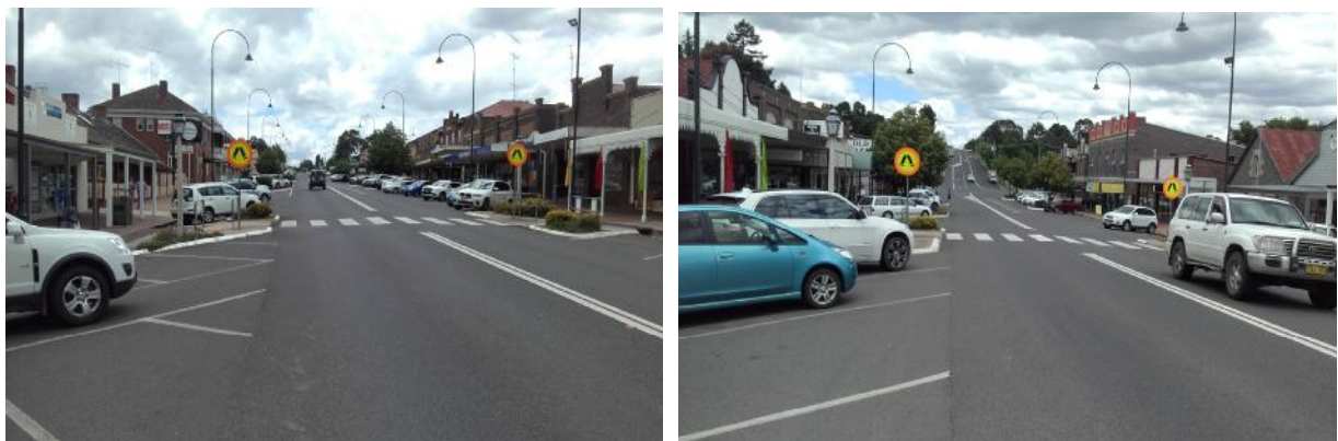
Fig 13 & 14. Southern and northern approaches to the Bridge Street Pedestrian Crossing. Southern approach has clear sightlines as driveway with no parking adjacent. Northern is concealed by parked cars protruding toward the traffic lanes, due to the 200mm high kerb at rear, proposed to be resolved.
