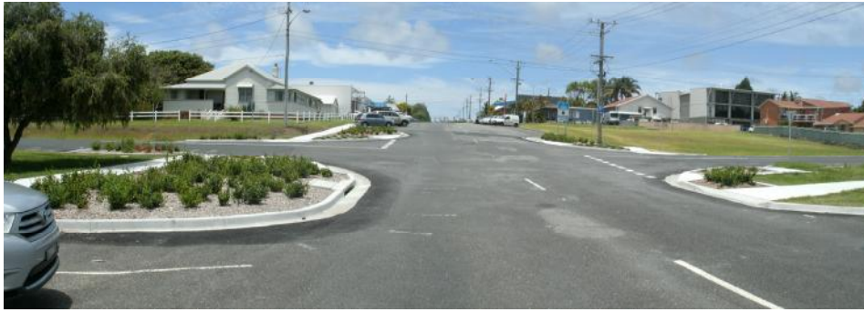
Fig 7. Example of Closed-in Intersection with shorter pedestrian crossing distances, holding-lines moved forward, enclosing the traffic. – Even though this street needs trees.
