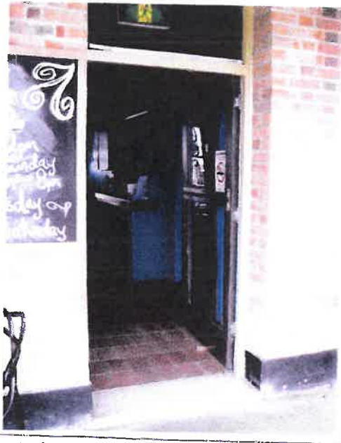
MAIN ENTRY DOOR. 35 MM THRESHOLD OFF FRONT VERANDAH
