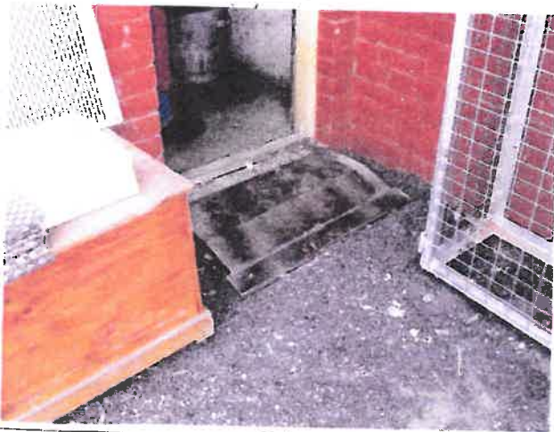
WALL TO BE EXTENDED TO GAS BOTTLE ENCLOSURE & NEW DOOR TO PROPOSED UNISEX TOILET ON NORTH SIDE.
