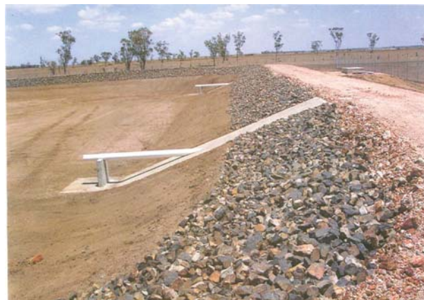
Typical Oxidation Pond Construction (Boggabilla)
