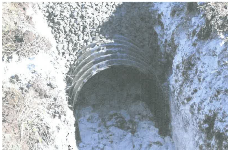
Figure 6 Liming/gypsum spreading in trench
