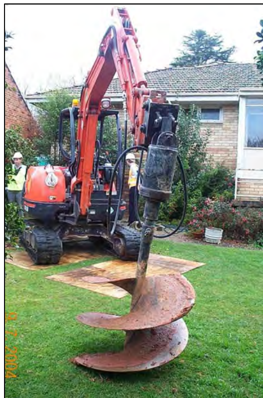
Typical Excavation for Low Pressure Pump Unit
