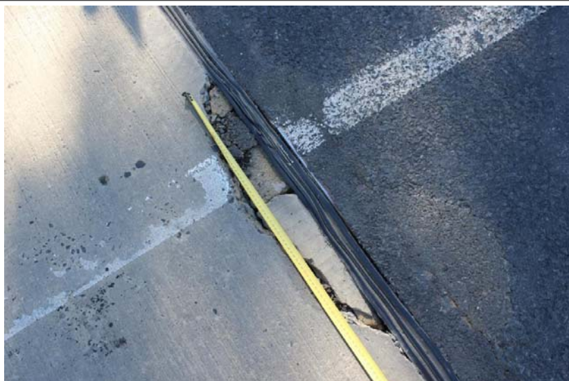
700mm long crack in centre deck at Abutment A
