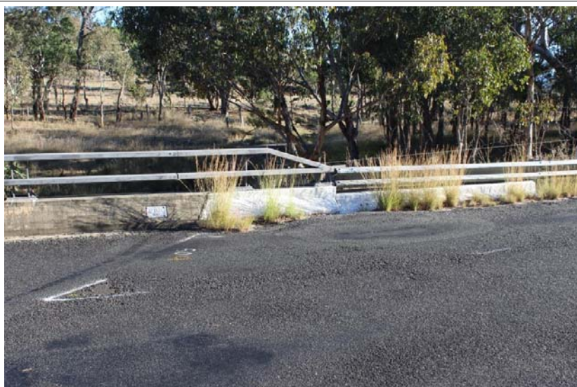
Settlement at Abutment A (northbound lane)
