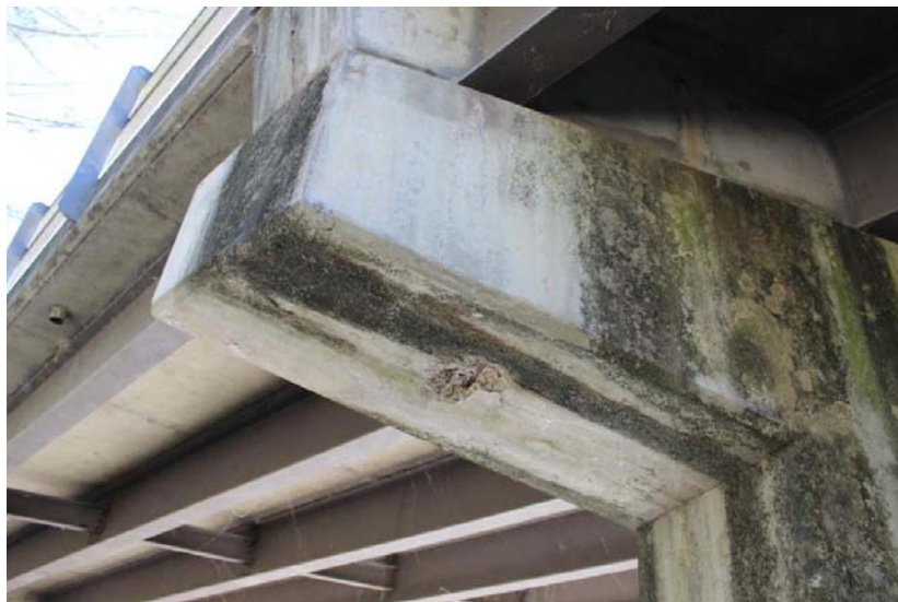
Spall at Pier 3
