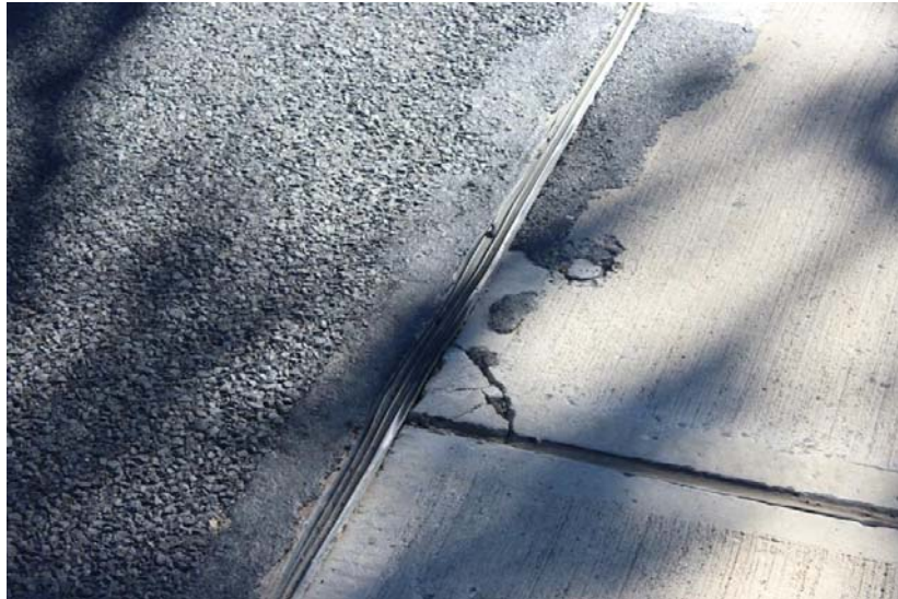
Cracked corner in centre deck at Abutment B
