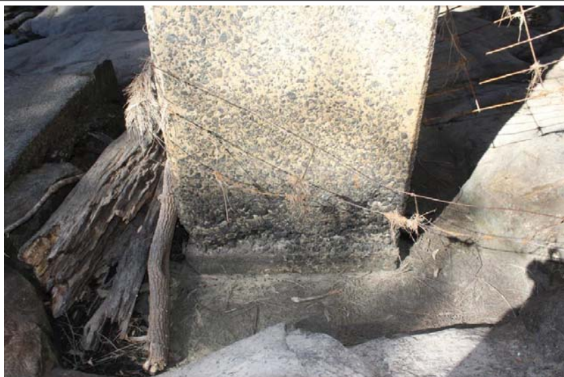
Weathering at pier column
