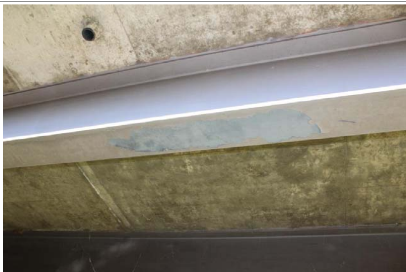
Loss of paint on beams
