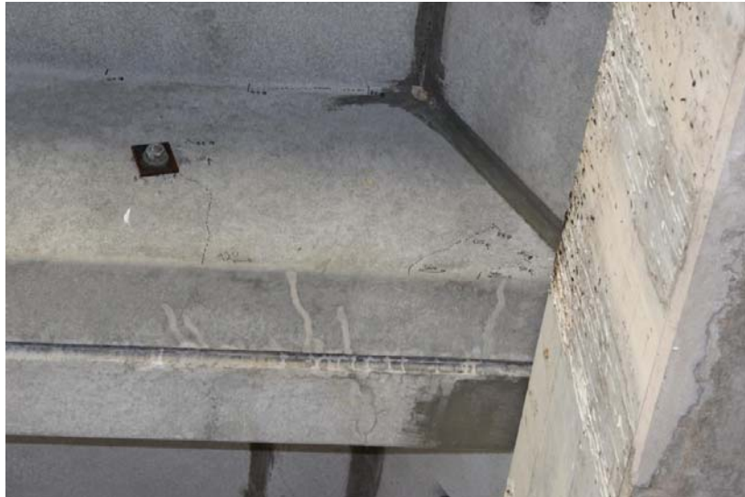
Span 2 flexural and shear cracking
