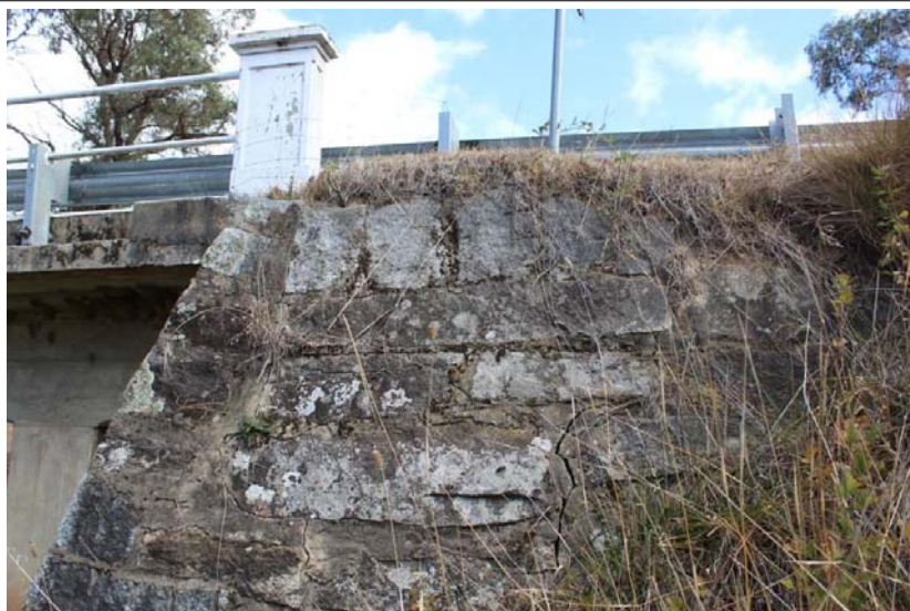
Crack in rock wall at Abutment B
