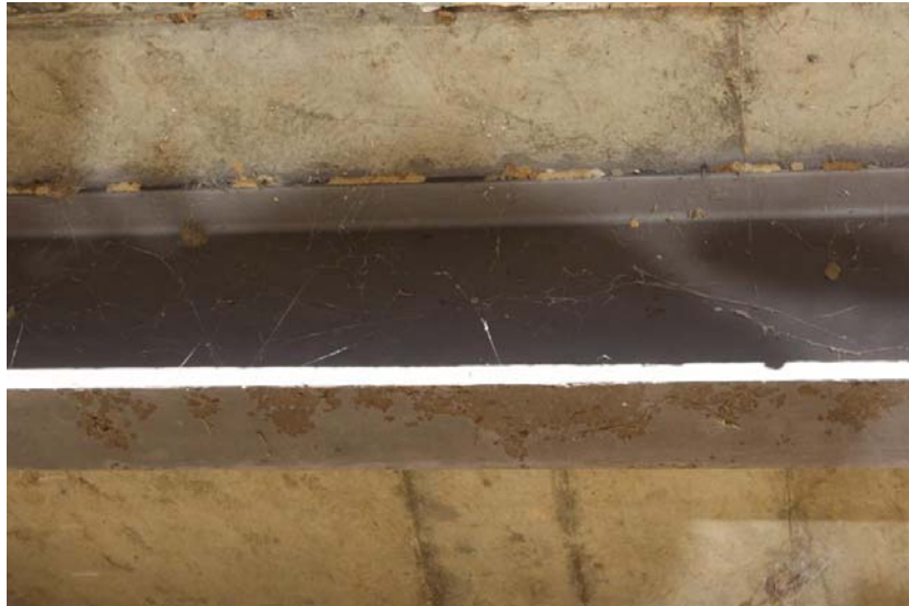
Minor corrosion in span 4 girder 6
