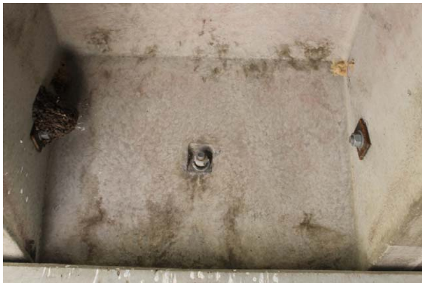
Loose tie bolt span 3 girder 5
