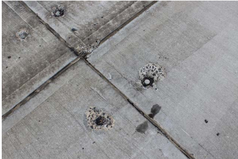
Spalling of deck concrete
