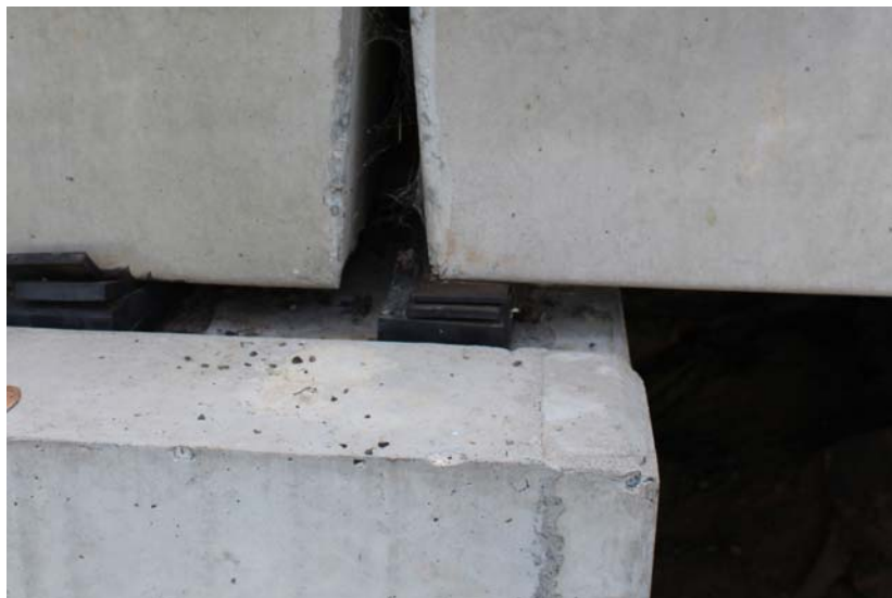
Bearing under downstream beam at Pier 3
