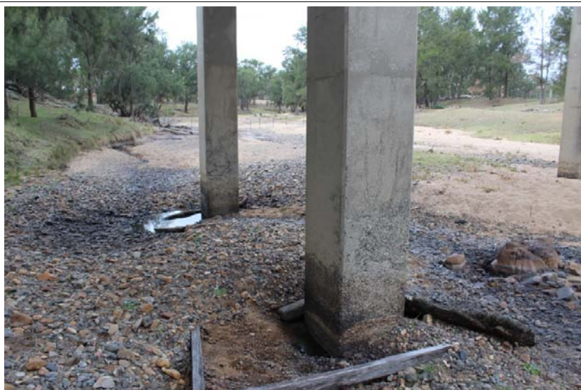
Loss of fines on pier columns
