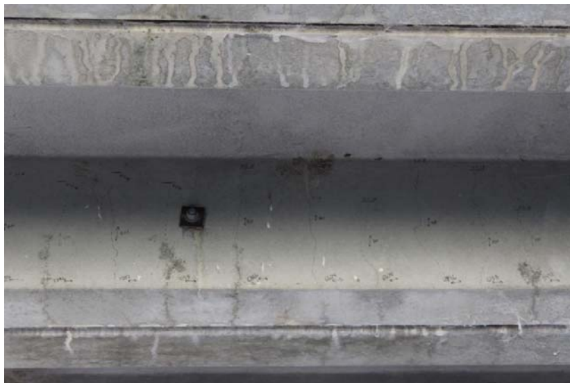
Span 2 flexural cracking
