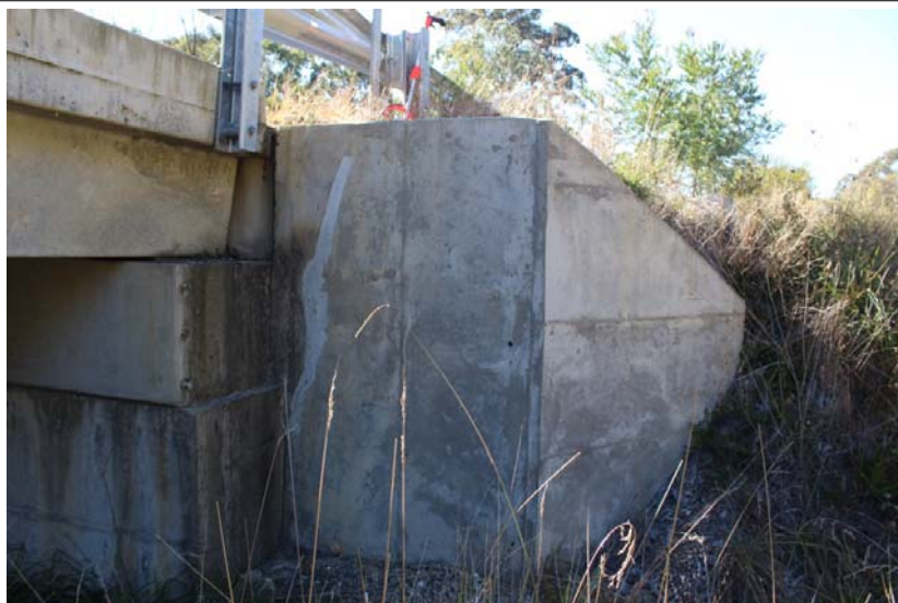
1mm crack in Abutment A wall (south side)
