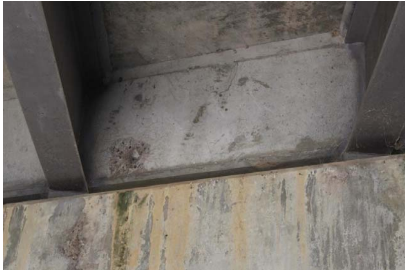
Spall in diaphragm at Pier 2
