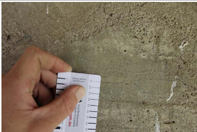
0.1mm horizontal crack in Girder 1 at Pier 1
