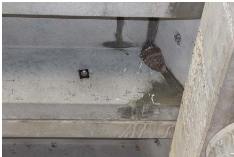
Span 2 flexural and shear cracking
