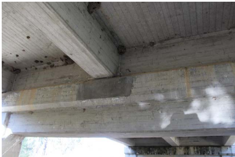
Repair to Pier 2 under Span 3 Girder 2
