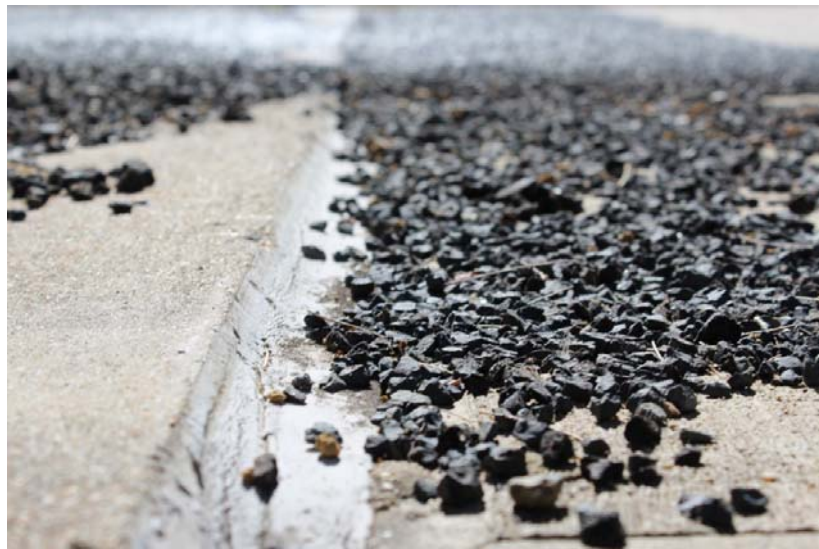
20mm difference between Abutment B and beams
