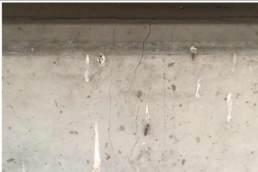
0.2mm vertical crack in Pier 3 headstock above upstream column
