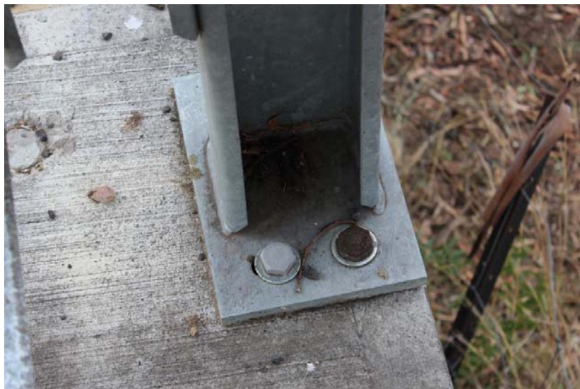
Non-galvanised barrier bolts
