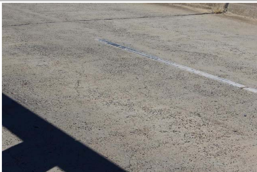
Cracking of deck surface
