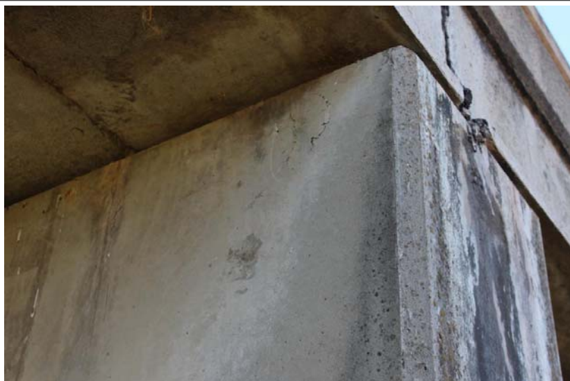
Spall on Pier 2 upstream
