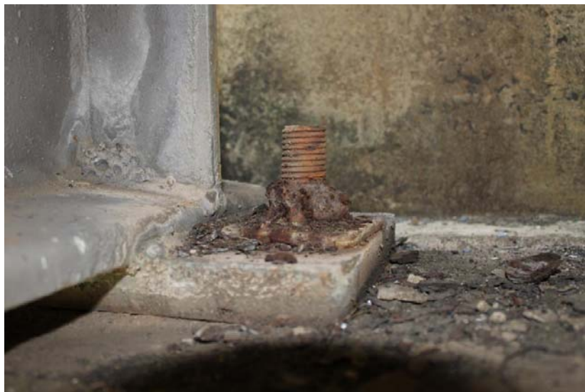
Corroded bearing bolts
