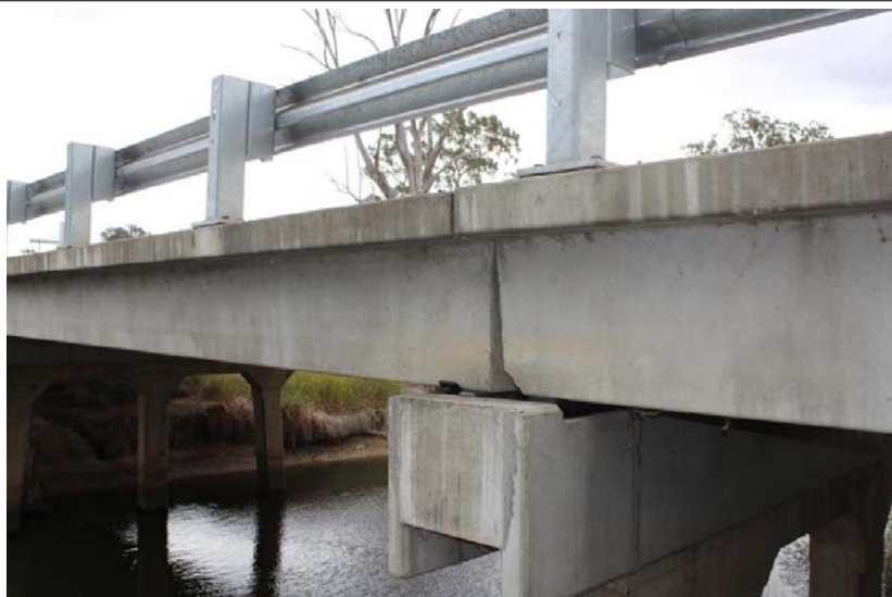
Pier 1 upstream and chipped corner on end of beam
