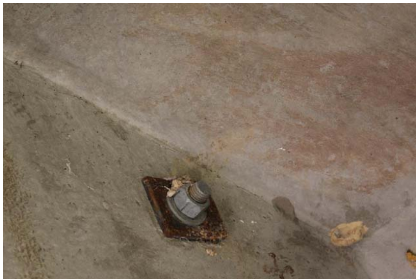
<0.1mm cracking at diaphragm and corroded plates on tie bolts
