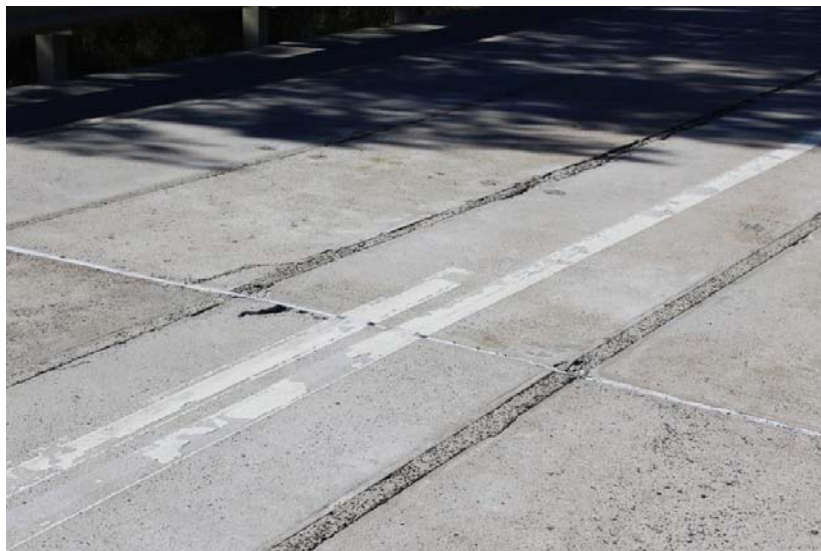
Chipping of beam ends
