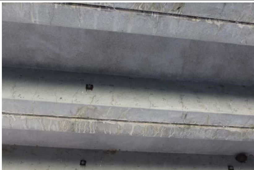
Span 2 flexural cracking
