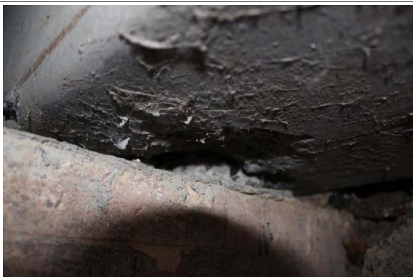
Spall in underside of span 4 beam 6 at Abutment B
